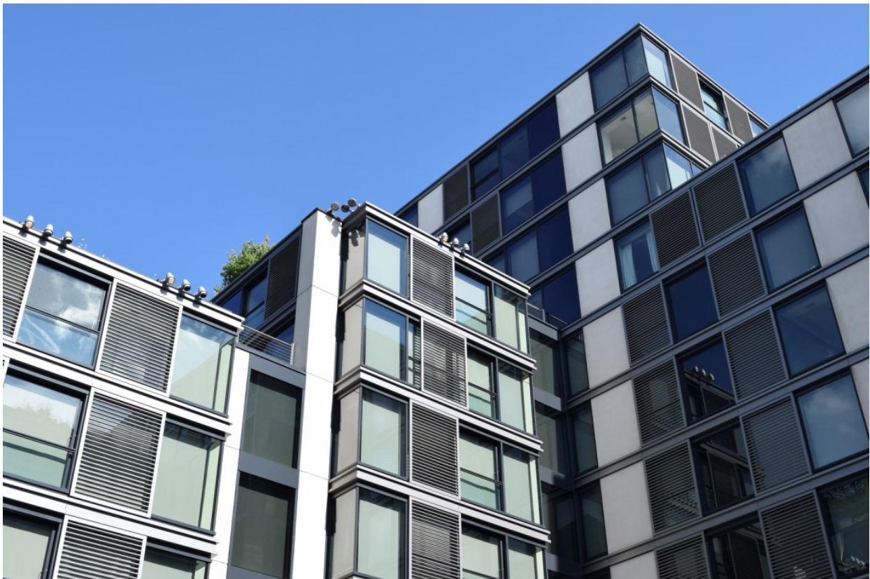
Figure 26 – Terraced floor counts allow for sunlight to reach the inner depths of the plaza.
