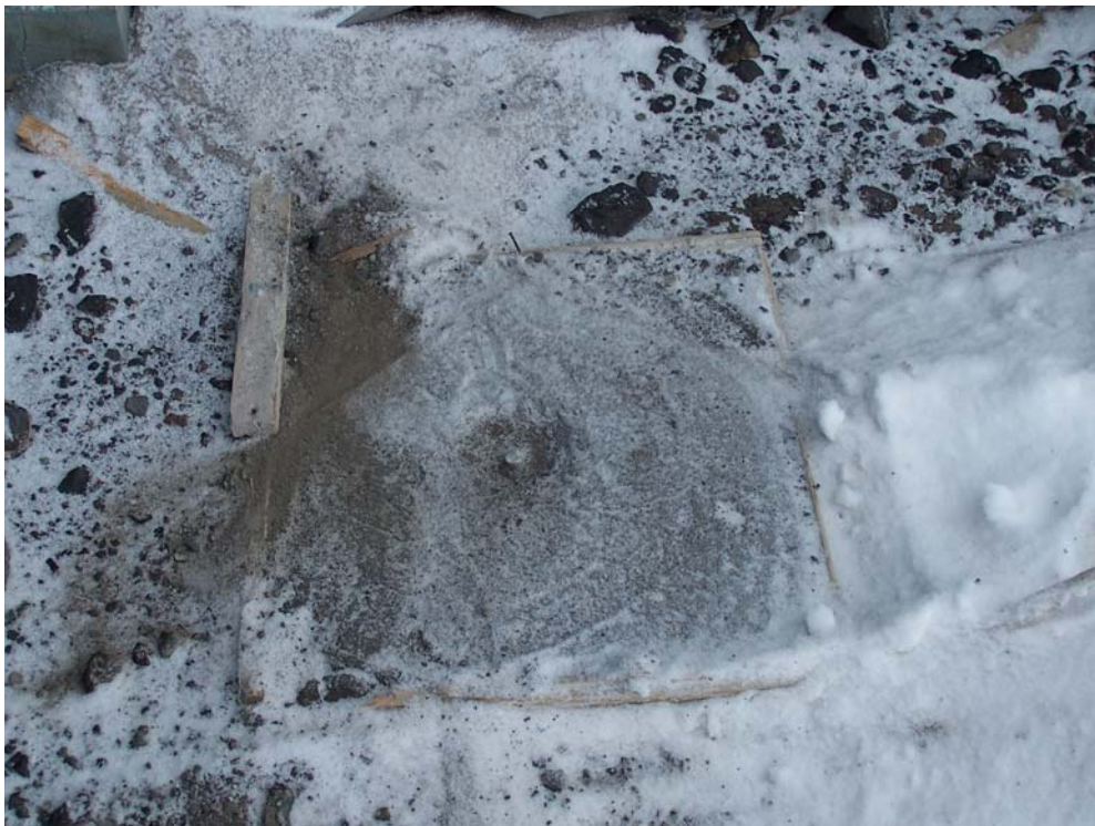
Figure 1.6: Metal pin in concrete slab on ground- assumed location of SEISMIC
