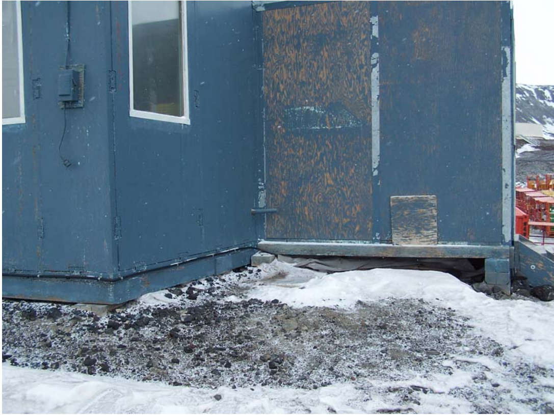
Figure 1.7: SE corner of Bldg. 139
