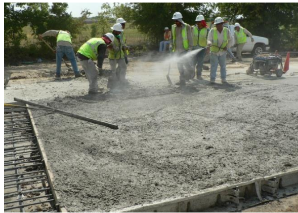
Figure 7.1 Placement of 100% manufactured sand sections (from personal collection)
