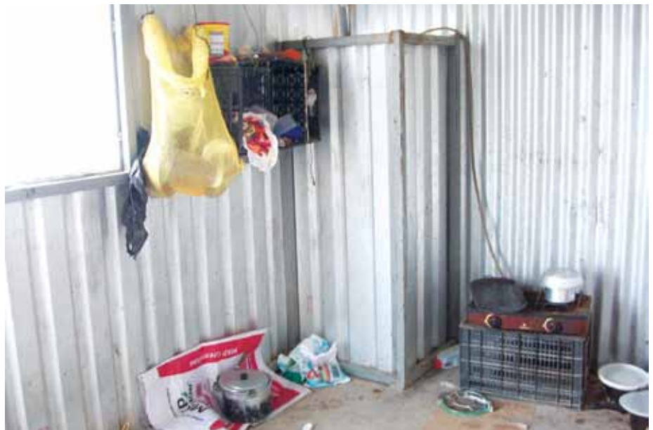
Type of housing provided by some invernaderos for workers.
