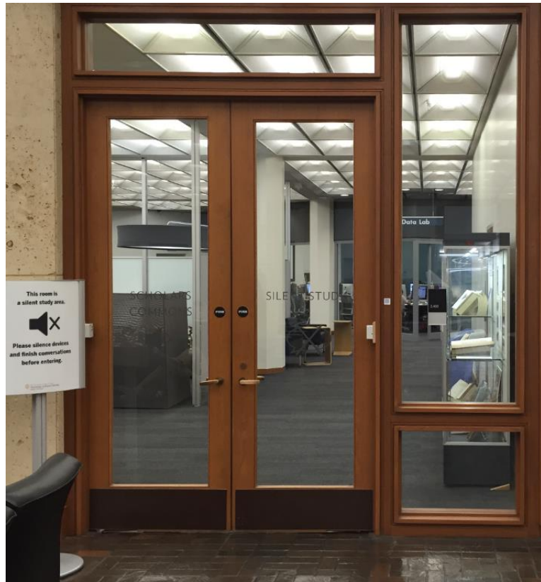
Prior to Blue Hanging Sign
