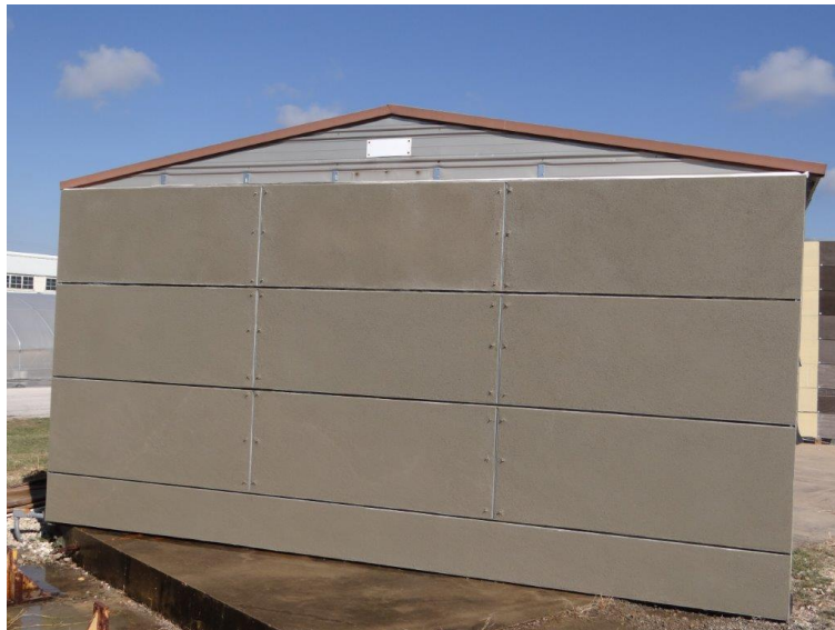
Figure 2.2: Stucco Wall at Completion.
