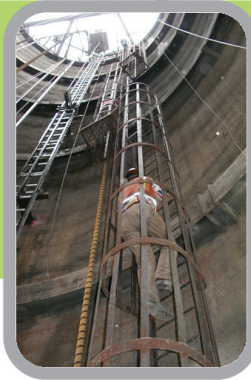
Tunnel shaft from below
