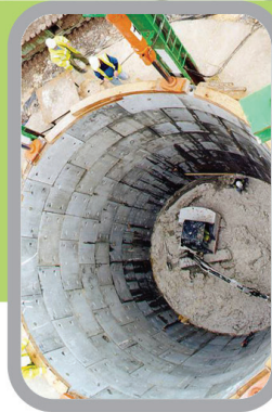
Tunnel shaft from above
