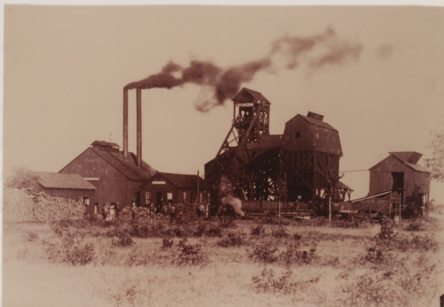
Figure 15. Tipple at mine site in Thurber, Erath County, Texas, about 1910. Mine was named "The Colonel." Wooden props stacked at left. (Photograph reproduced courtesy of Texas Highways Magazine, from negatives owned by Texas and Pacific Oil Company).
