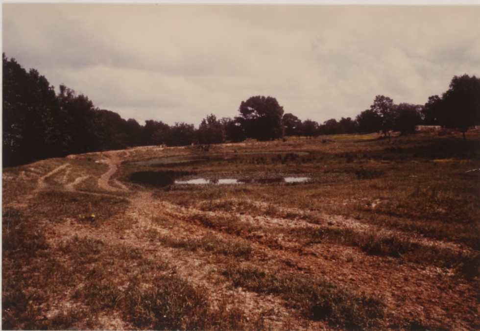
Figure 13. Area of subsidence at mine-site number Wd/A-1-2, Wood County, Texas, 1980. Site was reclaimed in 1980. Photograph by Deborah Kocurek, Railroad Commission of Texas (used with permission).
