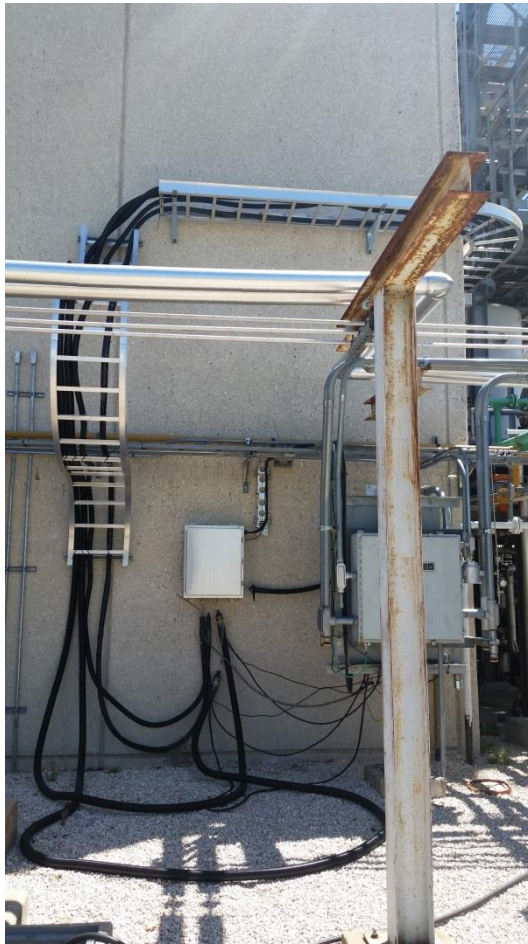
Figure C.14: Cable tray support and heated lines at termination at the MSSH
