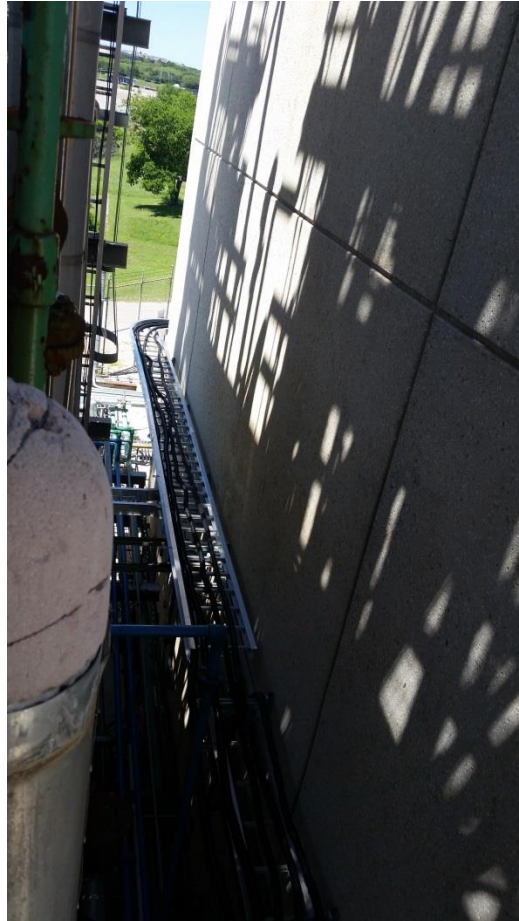
Figure C.11: Horizontal cable tray support for heated FTIR sample lines along south wall of CEER building
