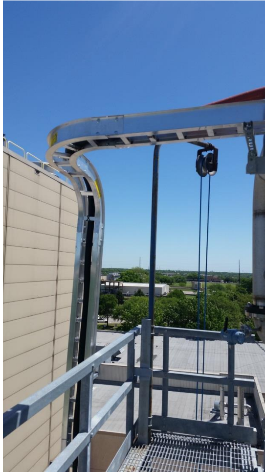
Figure C.12: Cable tray support and heated FTIR sample line for absorber outlet
