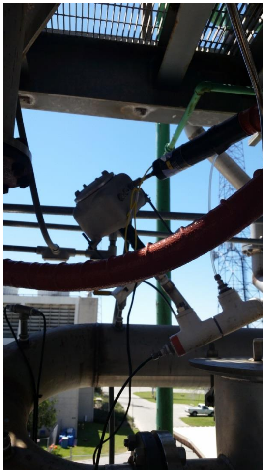
Figure C.7: FTIR sample probe at the knockout drum outlet
