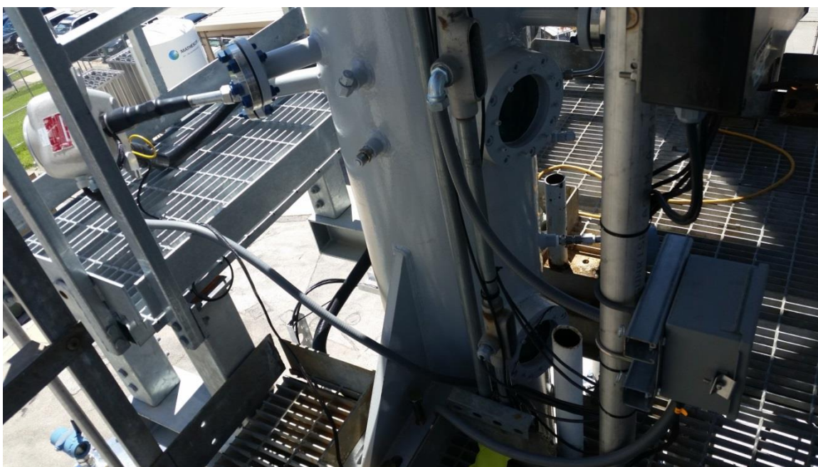
Figure C.5: FTIR sample probe between second and third stages of absorber. The box on the right contains terminal junctions for the FTIR probe and heated pad
