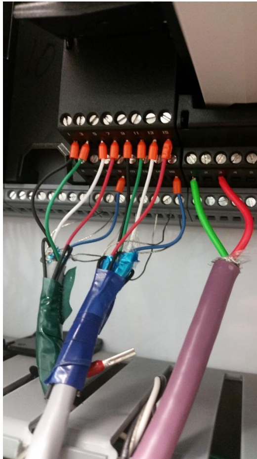
Figure C.18: RS-232 Terminal Block Pin Connections for FTIR to DeltaV™ Serial Communications Cable, at the DeltaV™ Terminal. The wire with the green tape is for the outlet FTIR, while the blue-taped wire is for the inlet.
