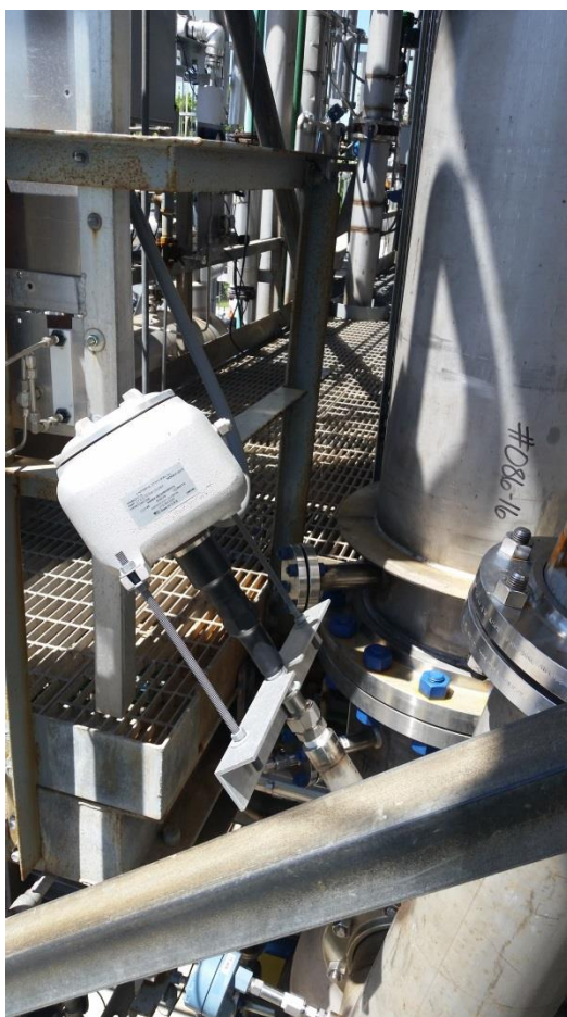
Figure C.3: FTIR Sample probe at absorber inlet
