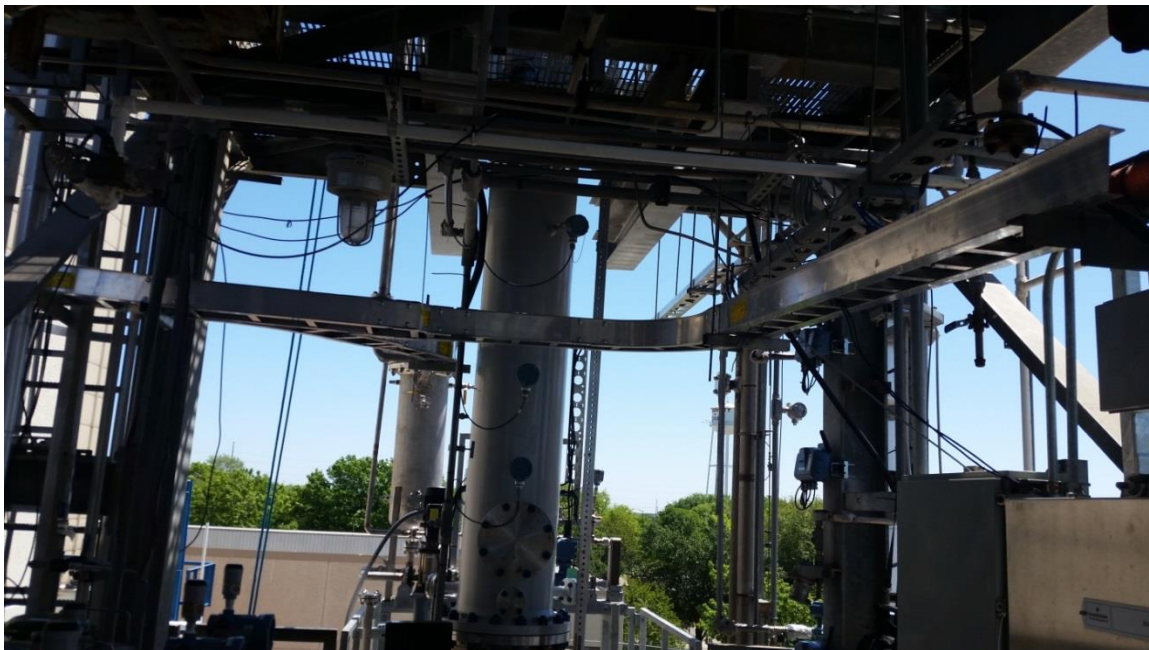
Figure C.9: Heated FTIR sample lines and supporting cable tray for absorber knockout drum and second/third stage sample locations
