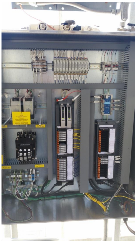
Figure C.8: Level 2 CHARMS box for heated pad and probe temperature control.
