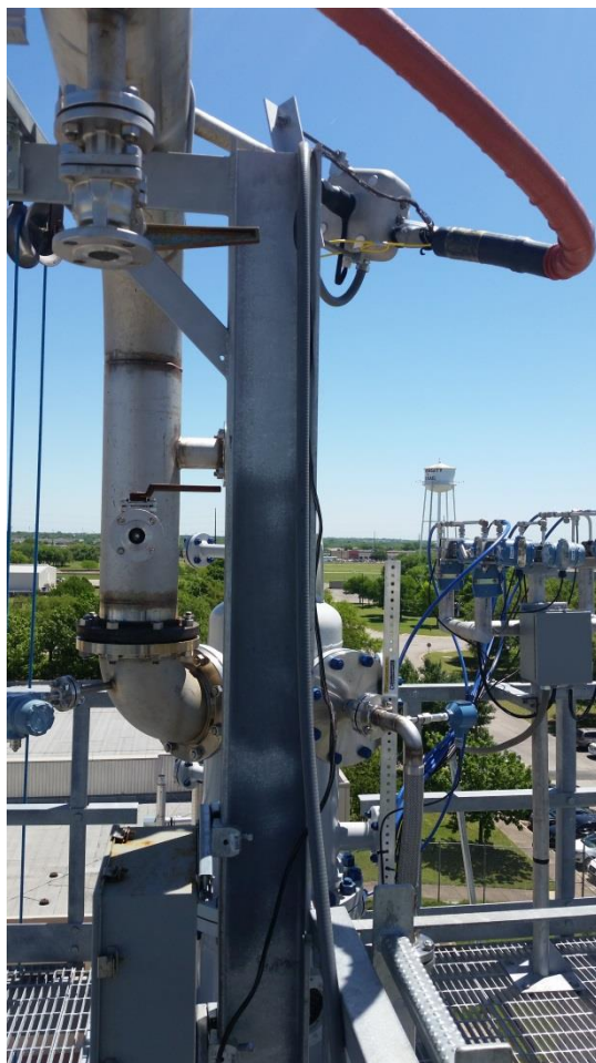
Figure C.6: FTIR sample probe at the absorber outlet. The box at the bottom of the picture contains terminal junctions for the FTIR probe and heated pad
