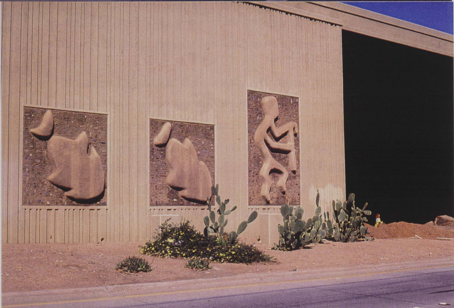
Figures 65 & 66: Typical Squaw Peak parkway overpass and retaining wall
