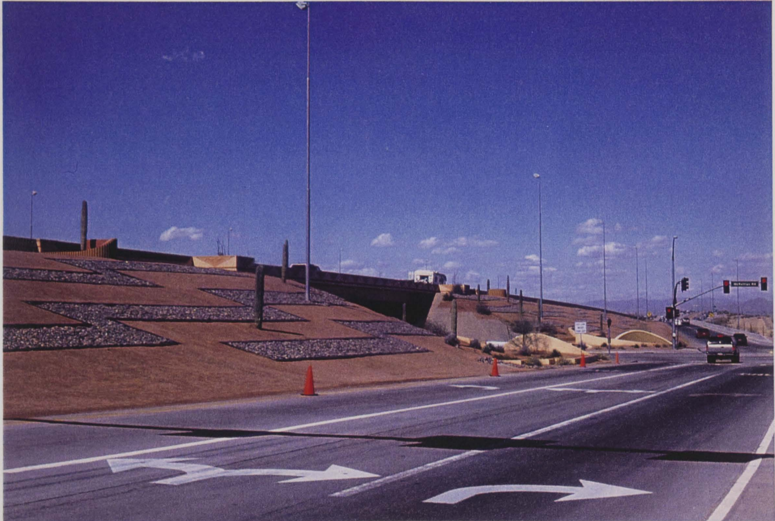
Figures 80 & 81: Pima freeway crushed aggregate embankment design treatments
