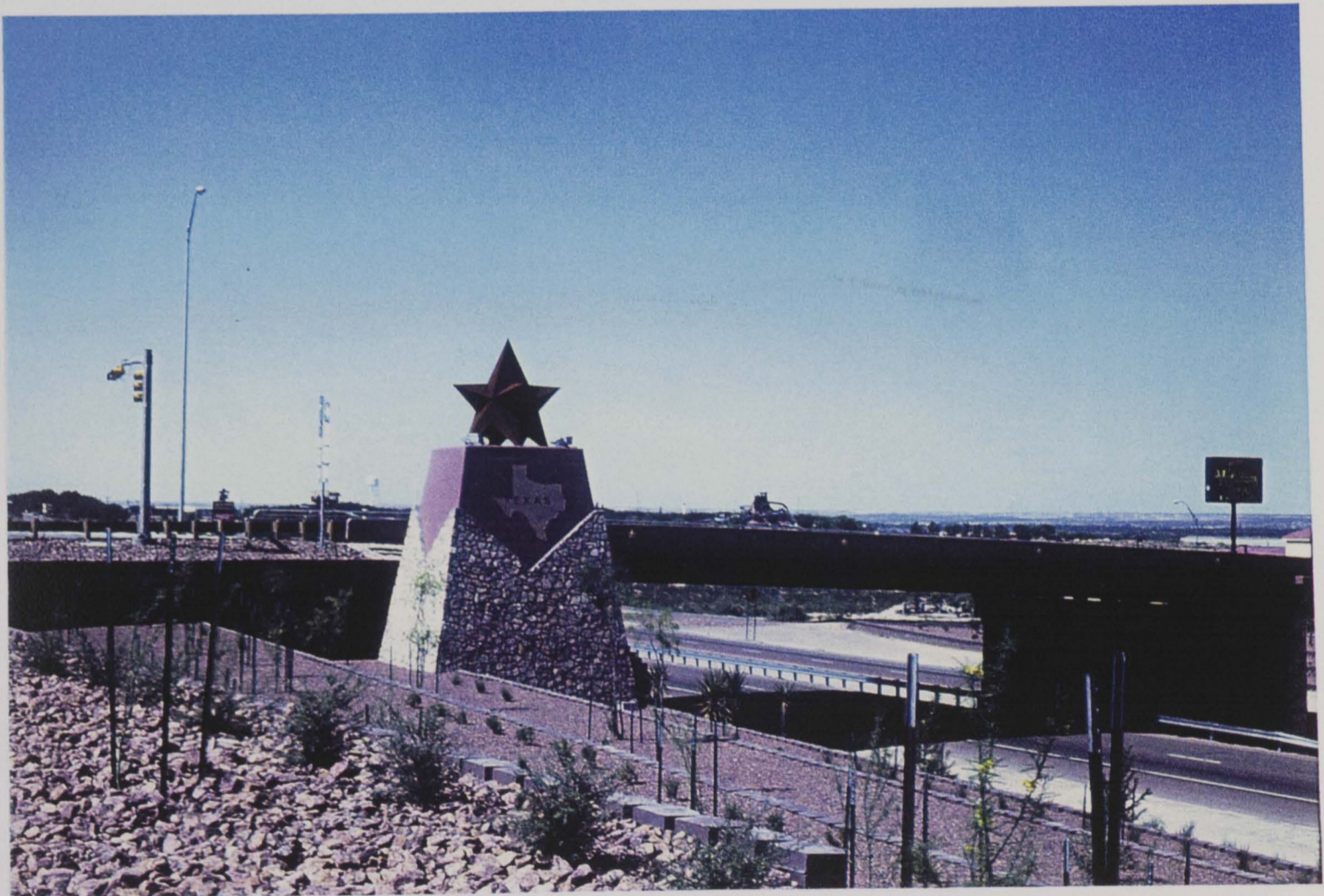
Figure 26: IH-10, Anthony, 1905 Bridge, New Mexico view
