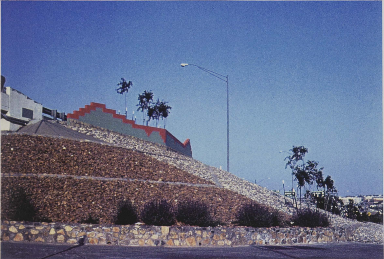
Figure 50 & 51: Examples of rehabbing exposed riprap slopes
