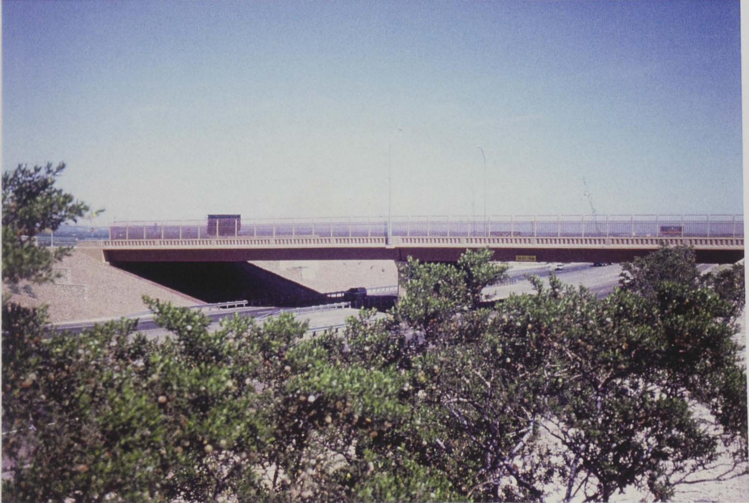
Figure 24 & 25: IH-10, Redd Road overpass and Artcraft Road overpass
