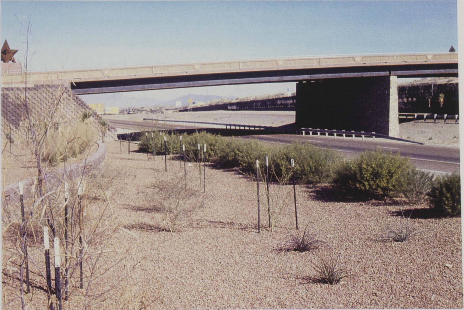
Figure 27 & 28: IH-10, Anthony Bridge, Texas views northward to New Mexico
