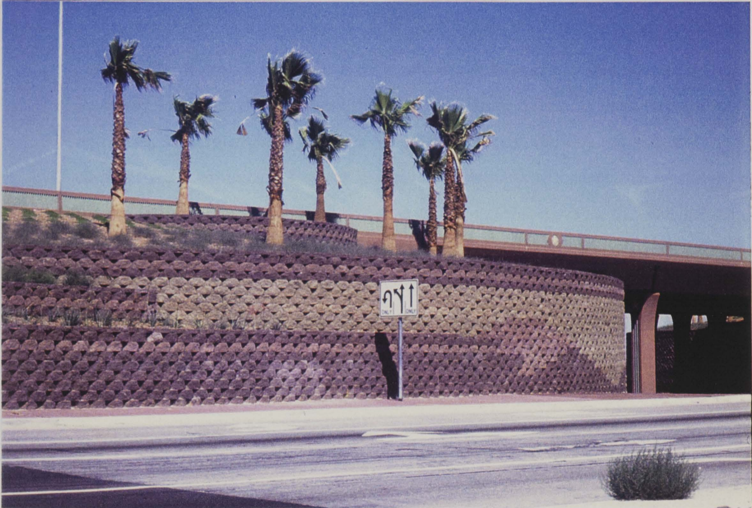
Figure 56 & 57: Fixed and loose stones, and concrete block retaining wall
