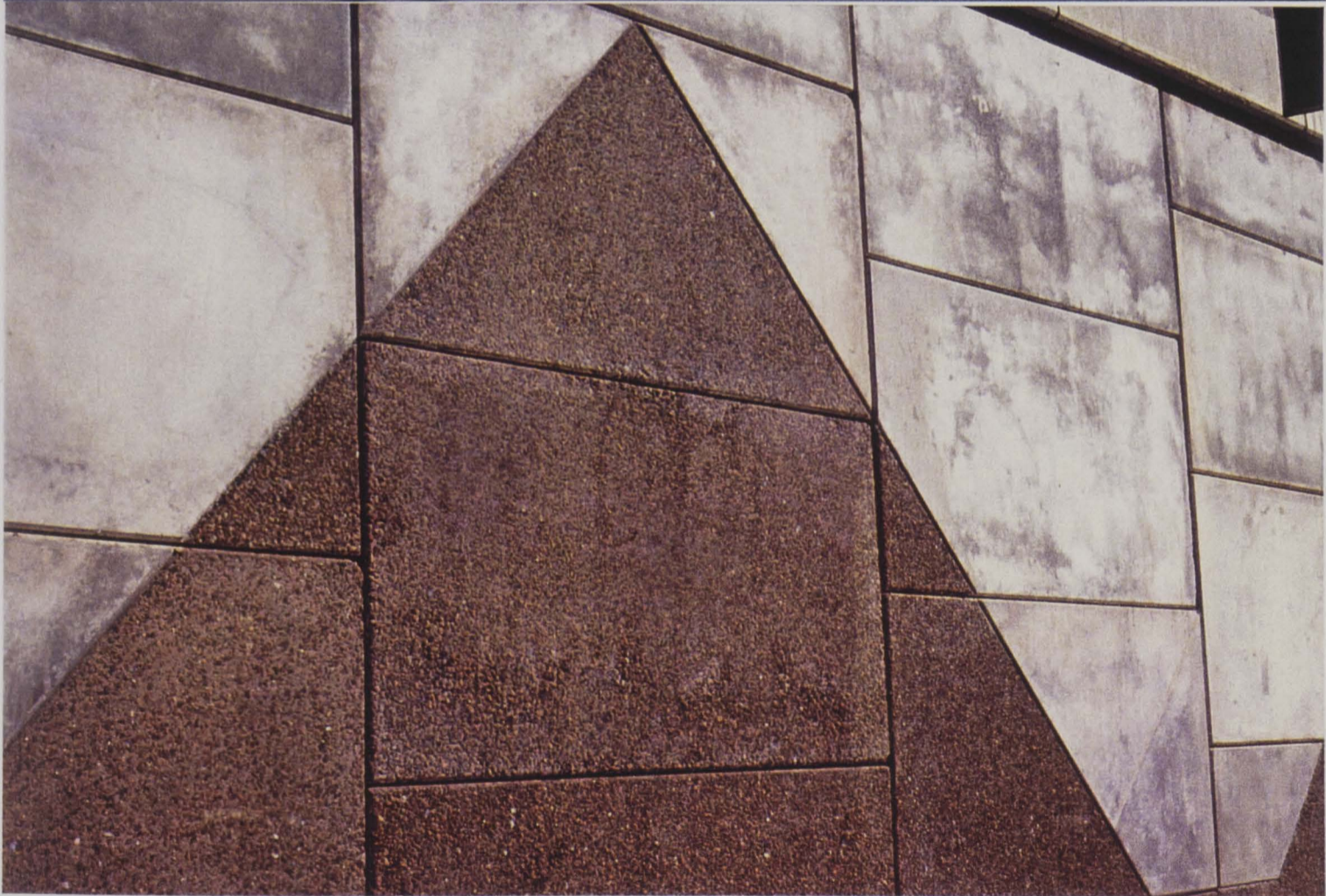
Figure 33 & 34: LP 375, Northeast, exposed aggregate retaining wall panels
