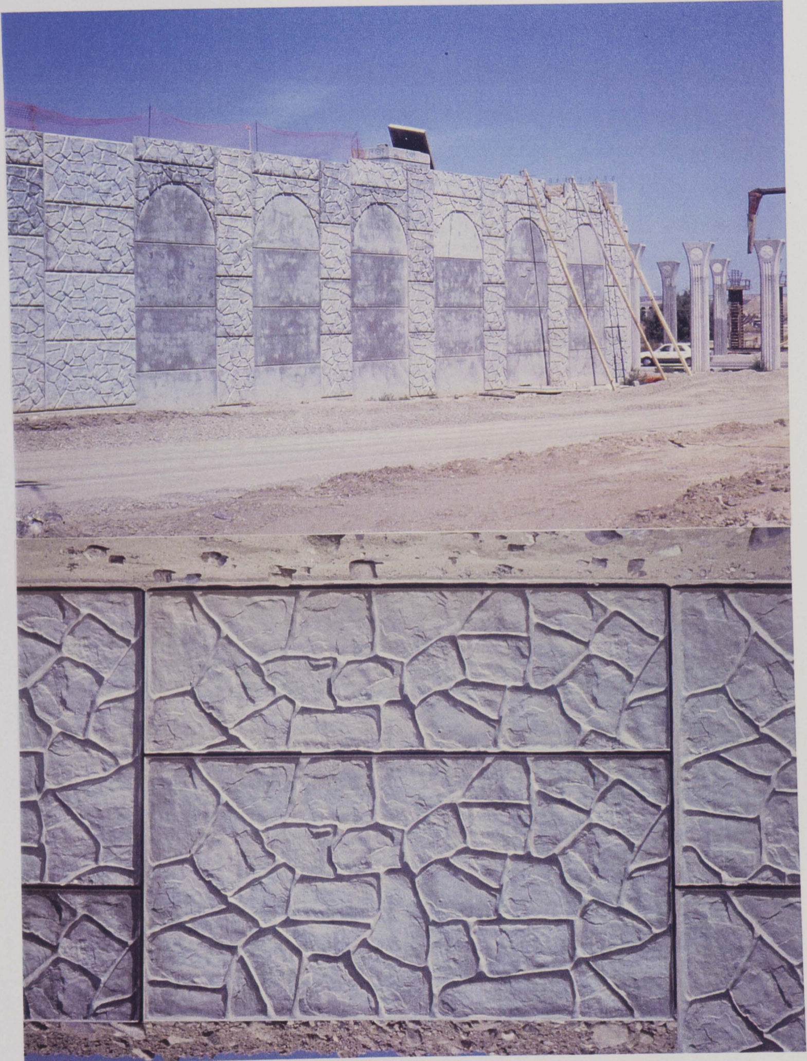
Figure 54 & 55: Artcraft Rd., custom form liners, using stone and arch patterns
