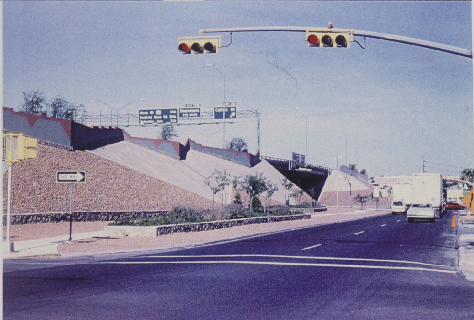
Figure 20 & 21: IH-10, before and after views of riprap embankments
