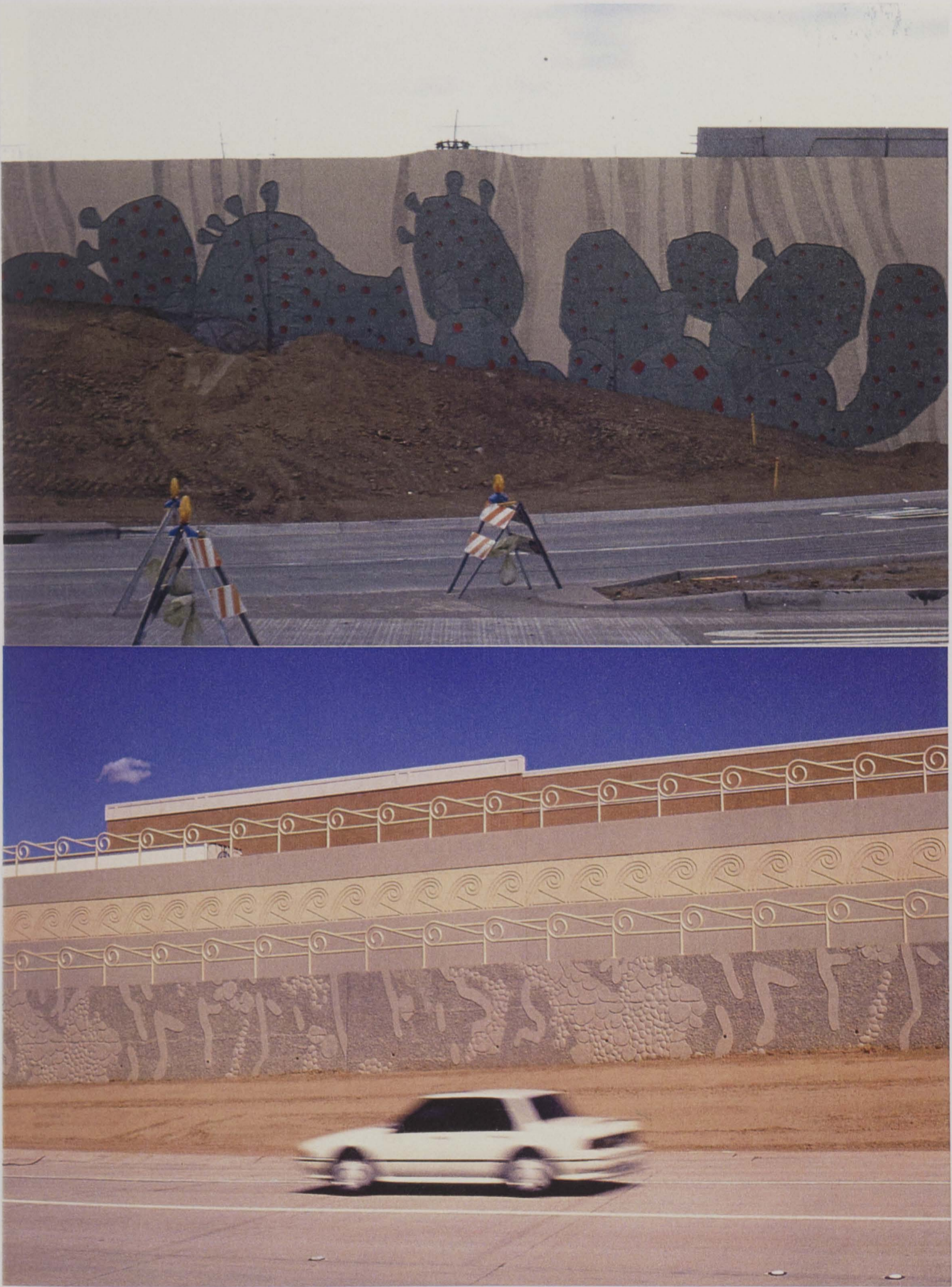
Figures 74 & 75: Pima freeway retaining walls in Scottsdale
