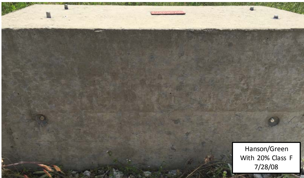
Figure 2: Precast plant exposure block replicate cast according to ASTM C1293 0.42 w/cm and 20% Class F fly ash
