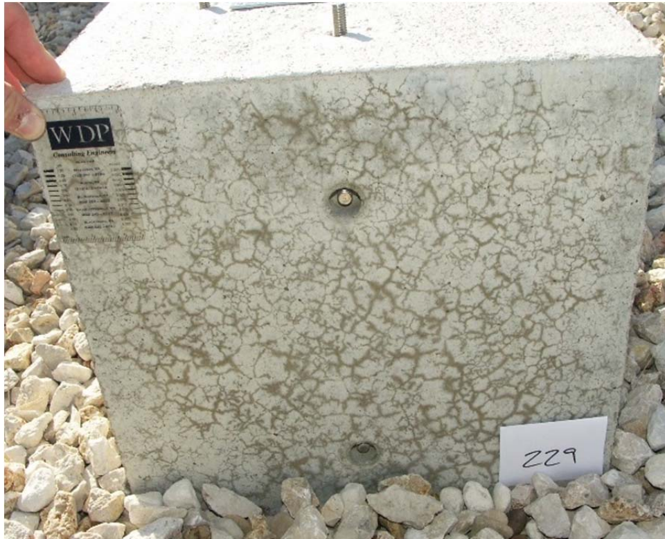
Figure 94: Example Crack Rating = 4.5
