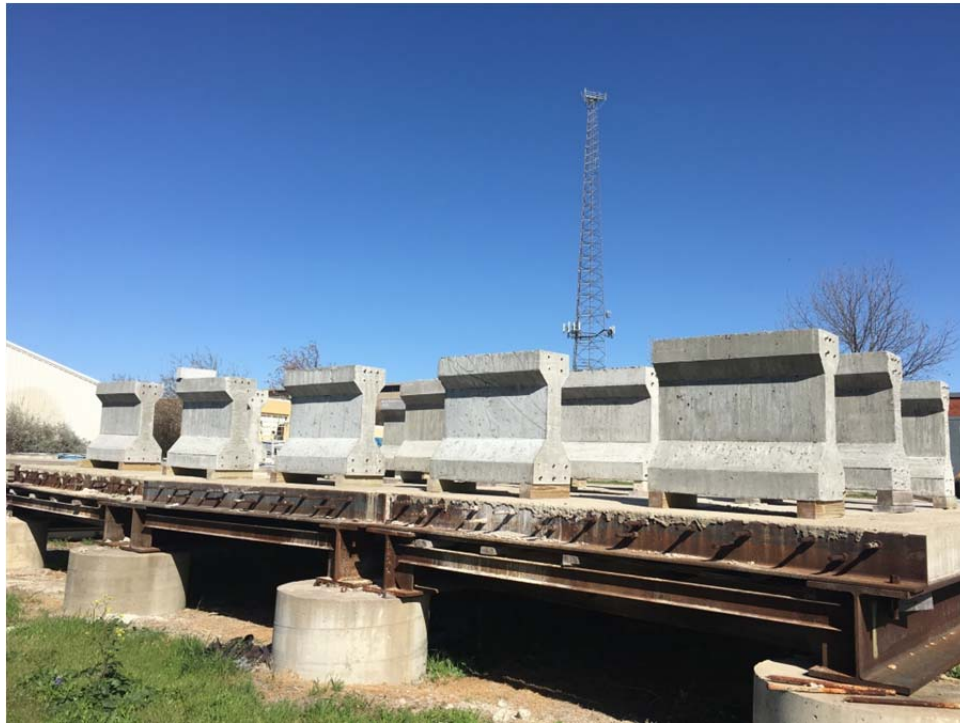
Figure 108: Mini Girder Exposure Site. Photo Taken Facing East.
