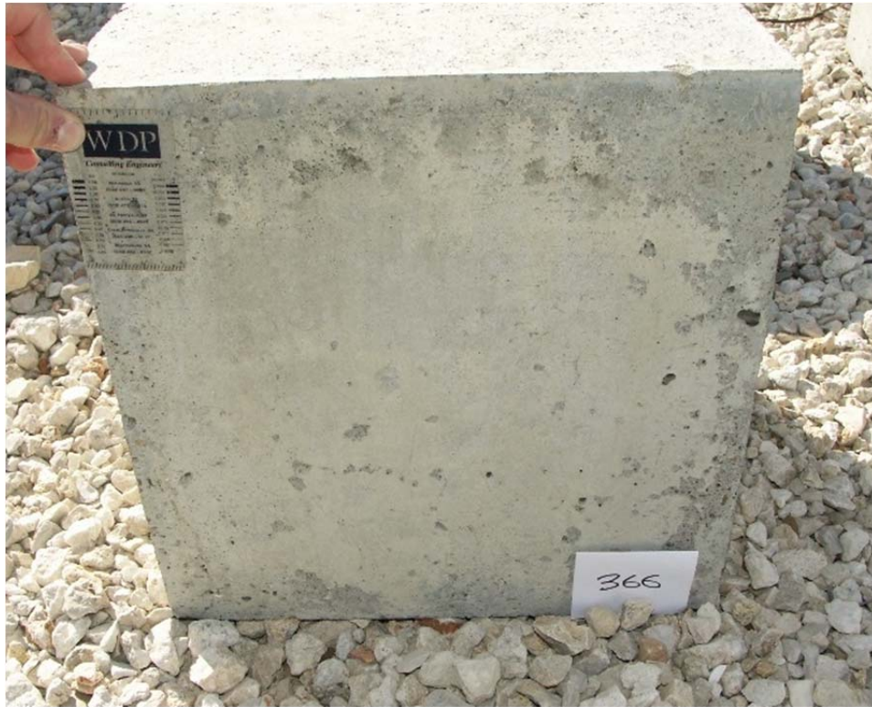
Figure 90: Example Crack Rating = 0
