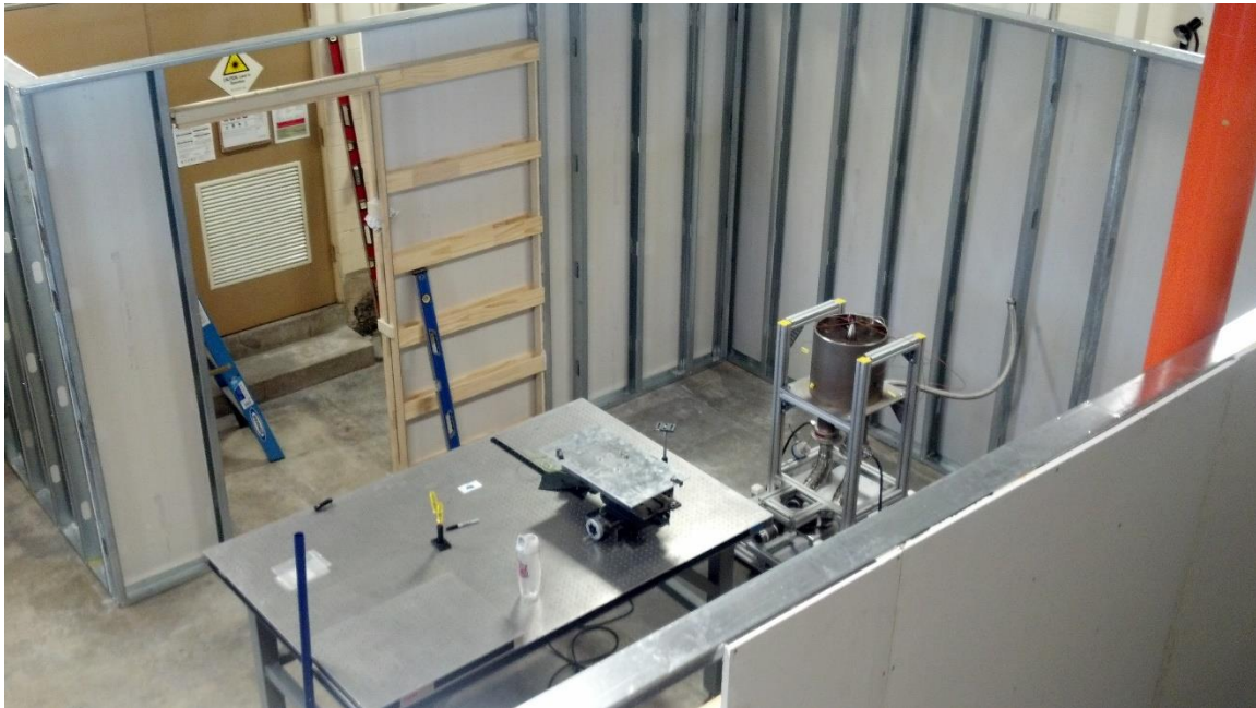
Figure A.1: Laser barrier walls being construction around facility
