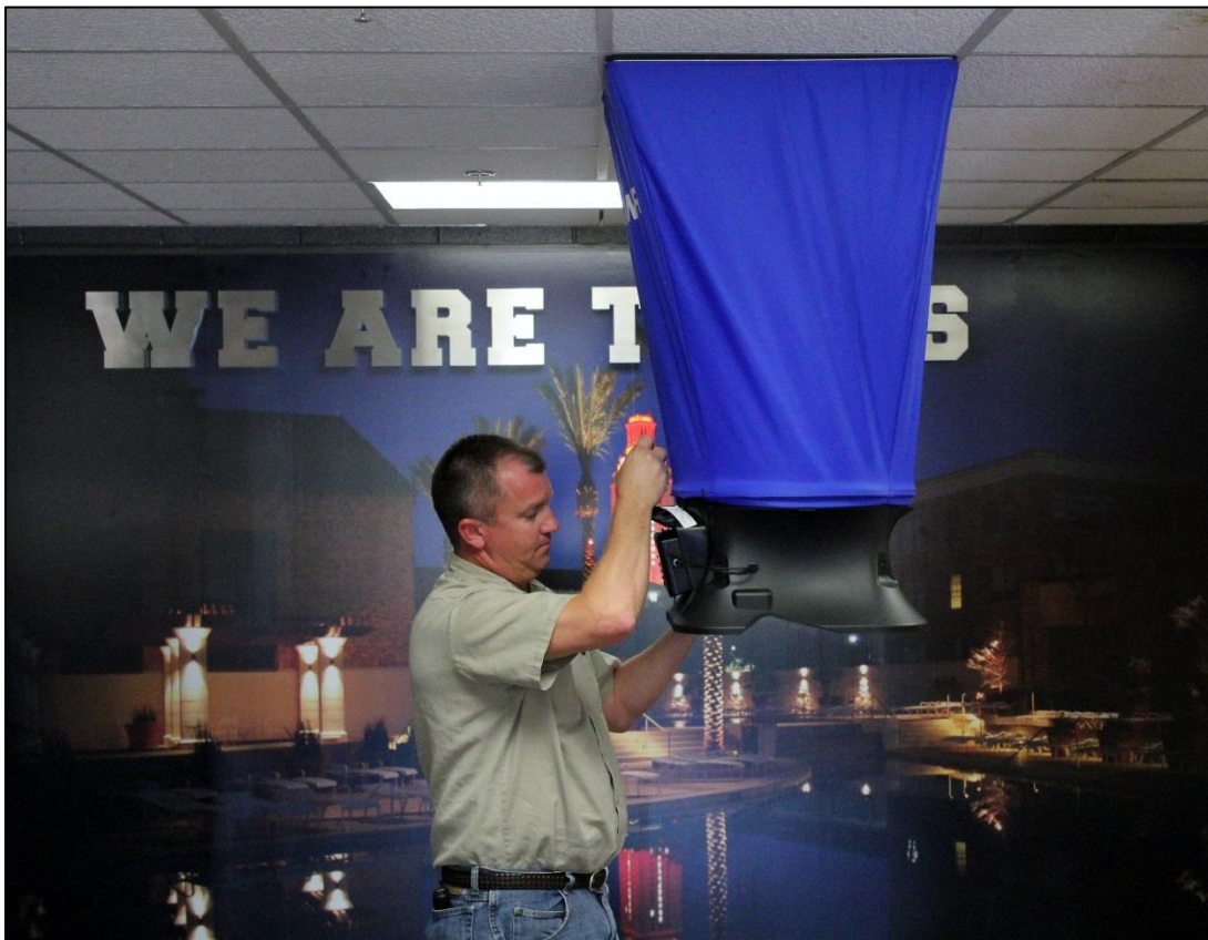
BOT technician performing audit of building systems.
