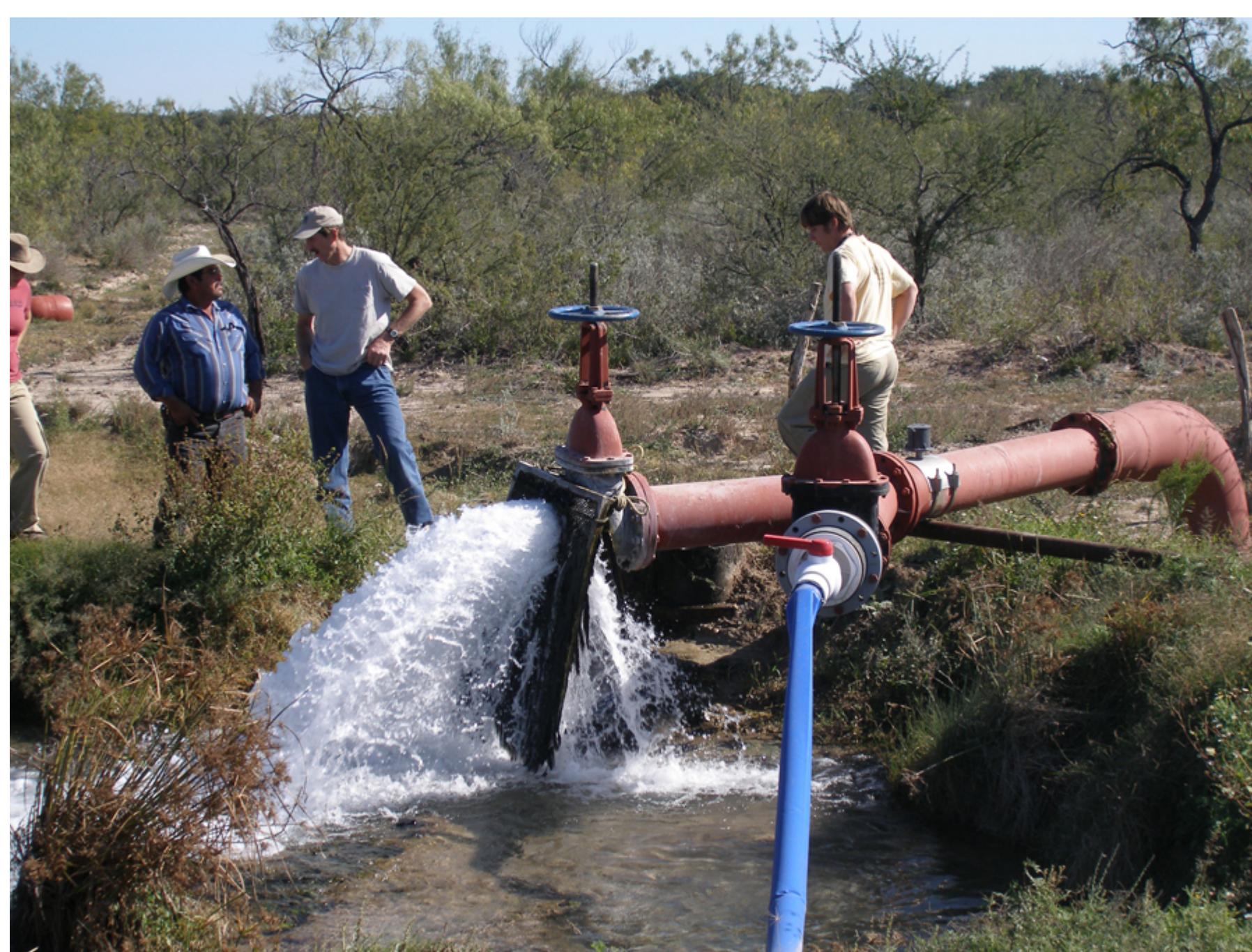
Artesian well at Rancho Veinticuatro, municipality of Zaragoza, Coahuila. Less permeable rocks at the surface confine water which can flow out under pressure when a well is drilled.
