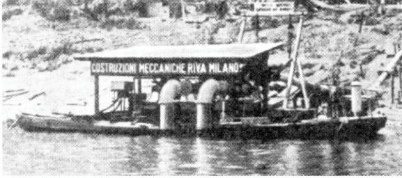
Mussolini's fascist government provided the resources that enabled excavators to drain Lake Nemi at the rate of about an inch per day. By June 1931, a little less than three years after the pumping began, an estimated 1.4 billion cubic feet of water had been removed from the lake. Il Duce visits pumping operations at Nemi, right
