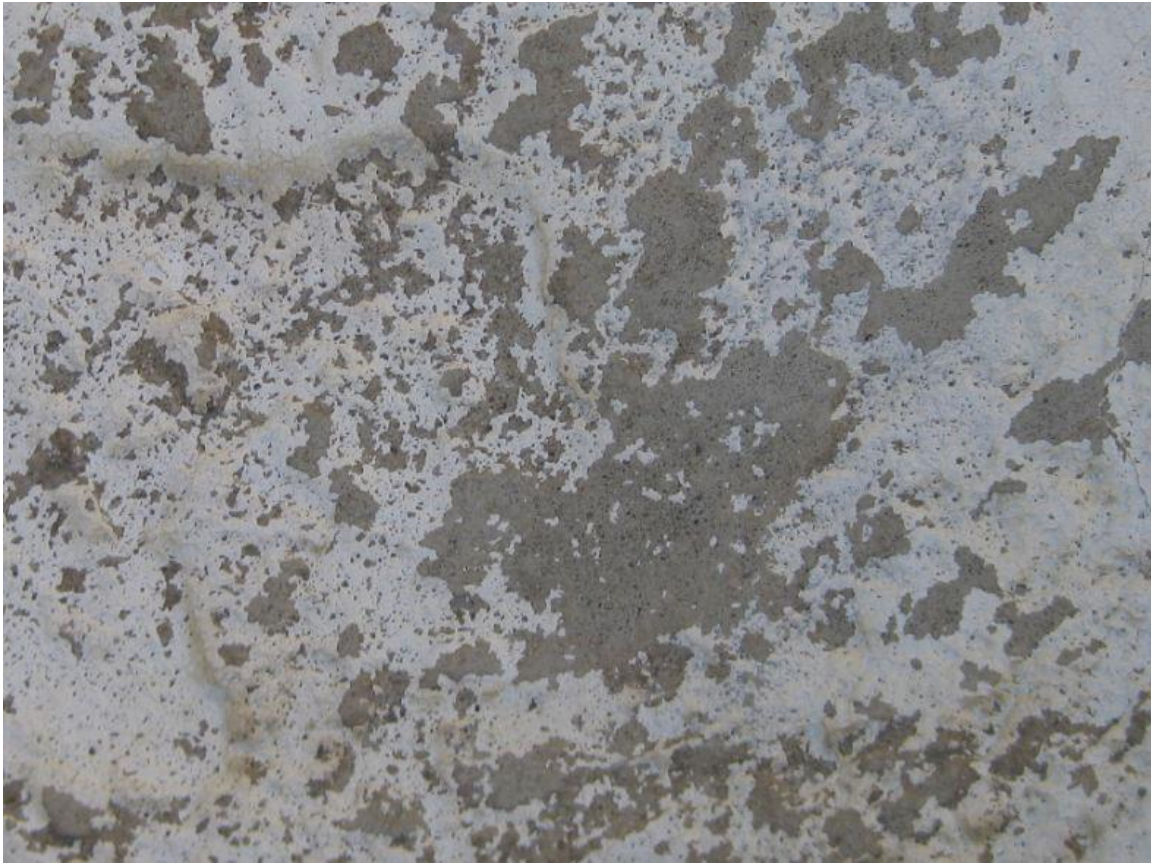
Figure 13: Cement stucco with aggregate visible.
