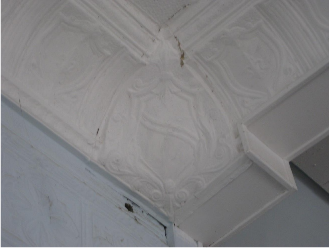
Figure 21: Detail of a pressed metal corner.
