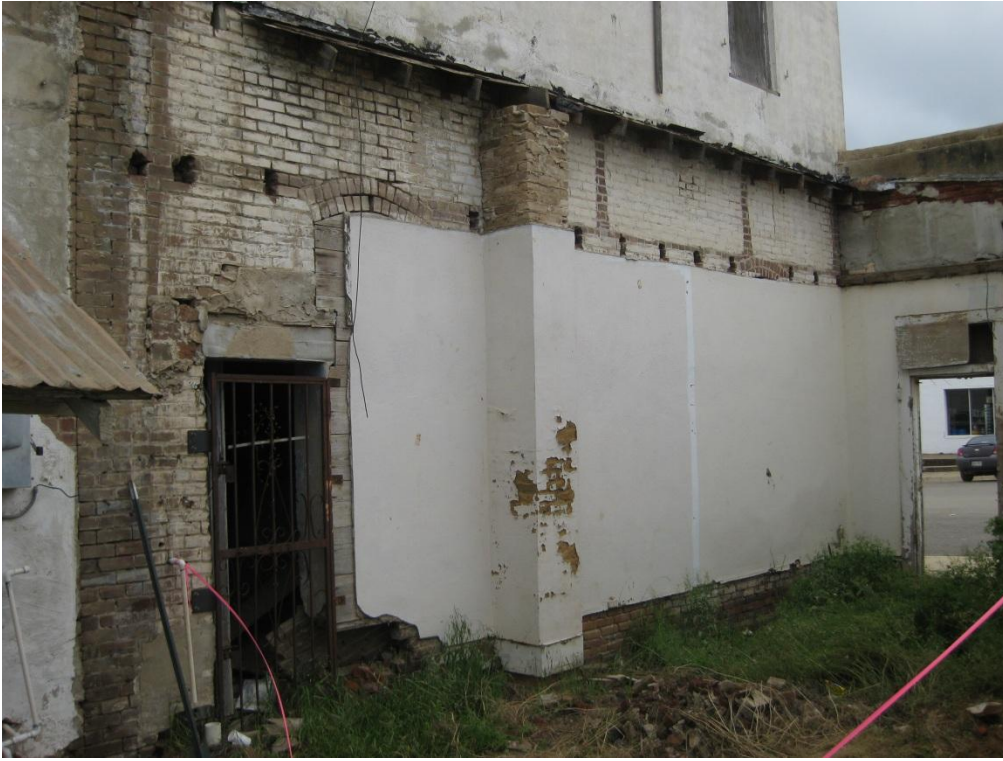
Figure 16: First floor of the Kerr Building's west elevation.
