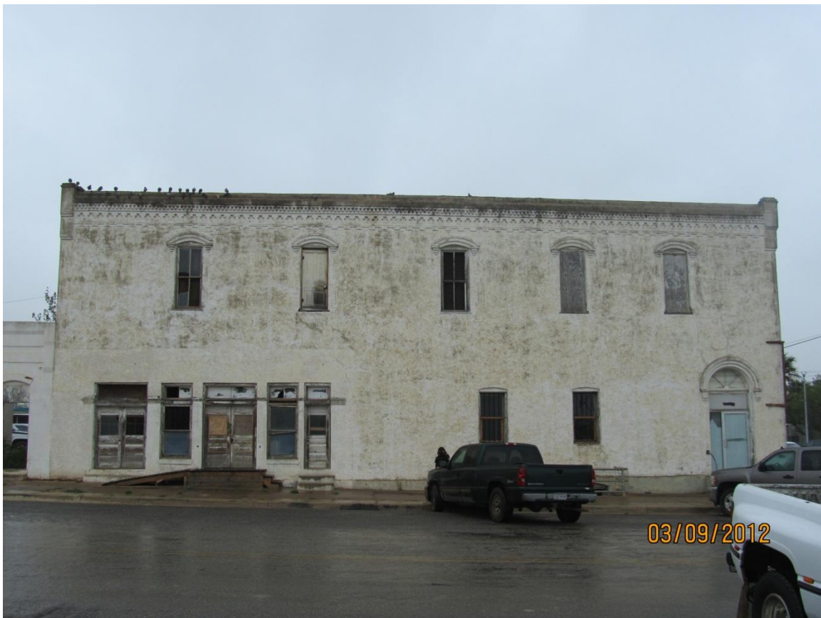
Figure 15: The south elevation of the Kerr Building.
