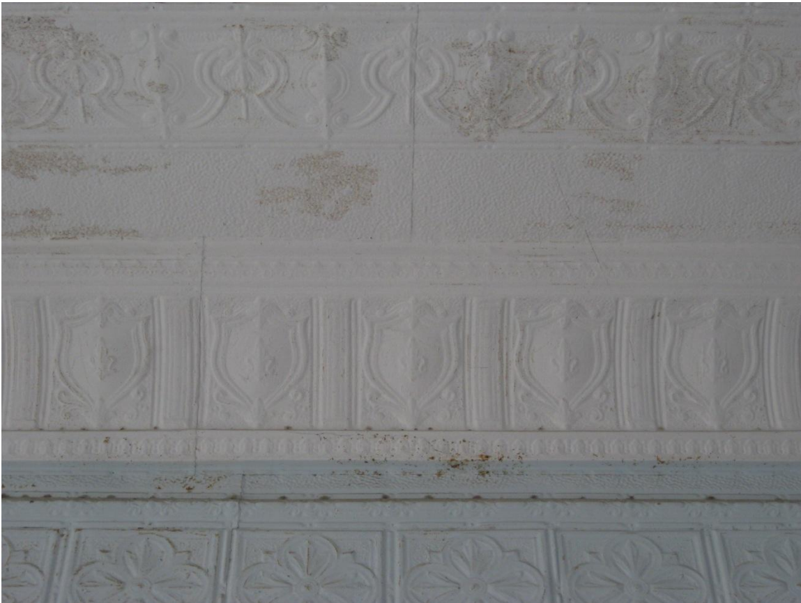
Figure 20: The transition from pressed metal wall to pressed metal ceiling.
