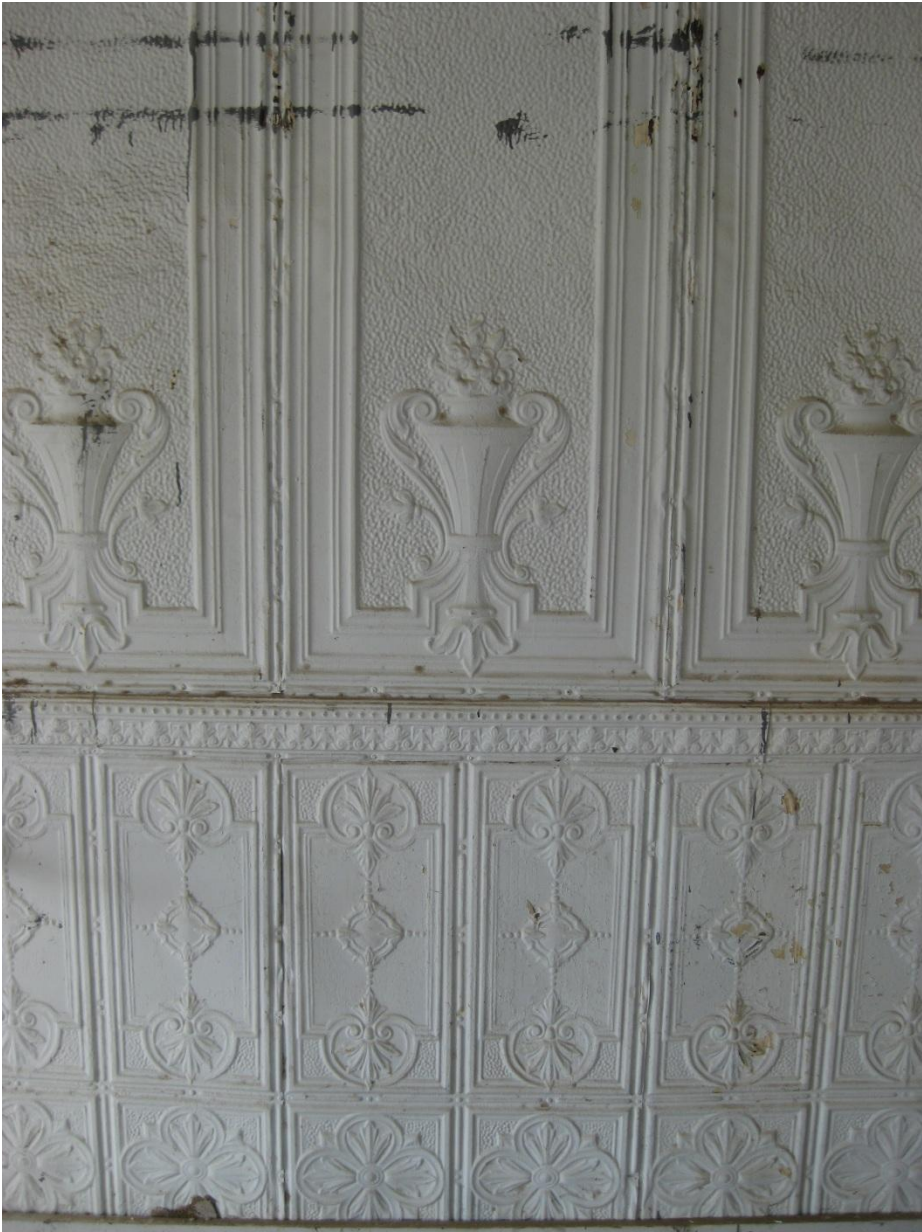
Figure 19: Lower portion of the pressed metal wall.
