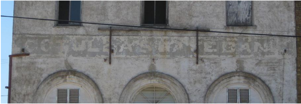
Figure 6: Painted sign on the façade of the Kerr Building. East elevation.
