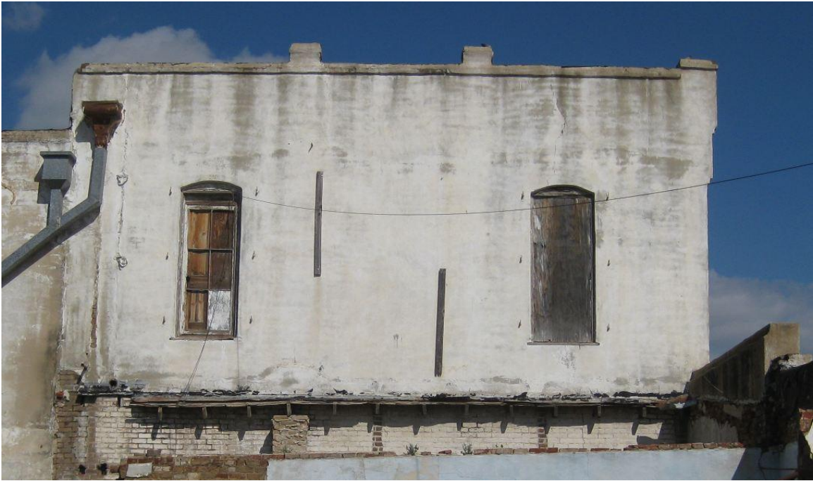
Figure 17: Second floor of the Kerr Building's west elevation.
