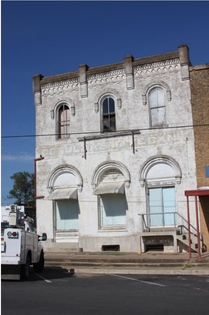
Figure 10: The Kerr Building in 2010. East elevation. (Source: Robert Mezquiti)
