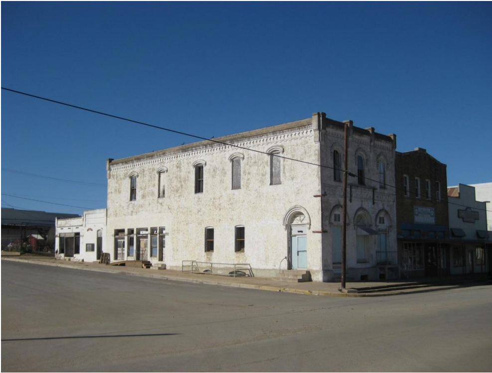
Figure 12: Overview of the Kerr Building. South and east elevations.
