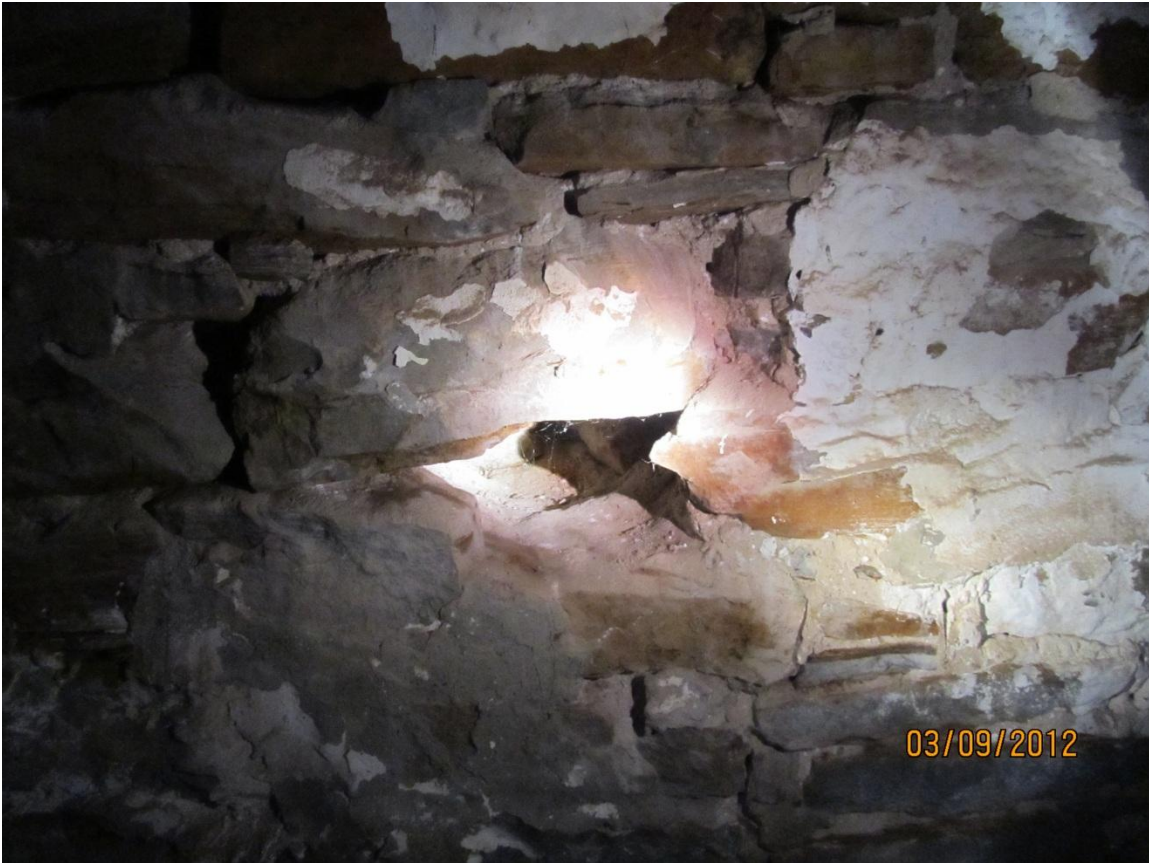
Figure 30: Coursed ironstone rubble on the basement's north wall.
