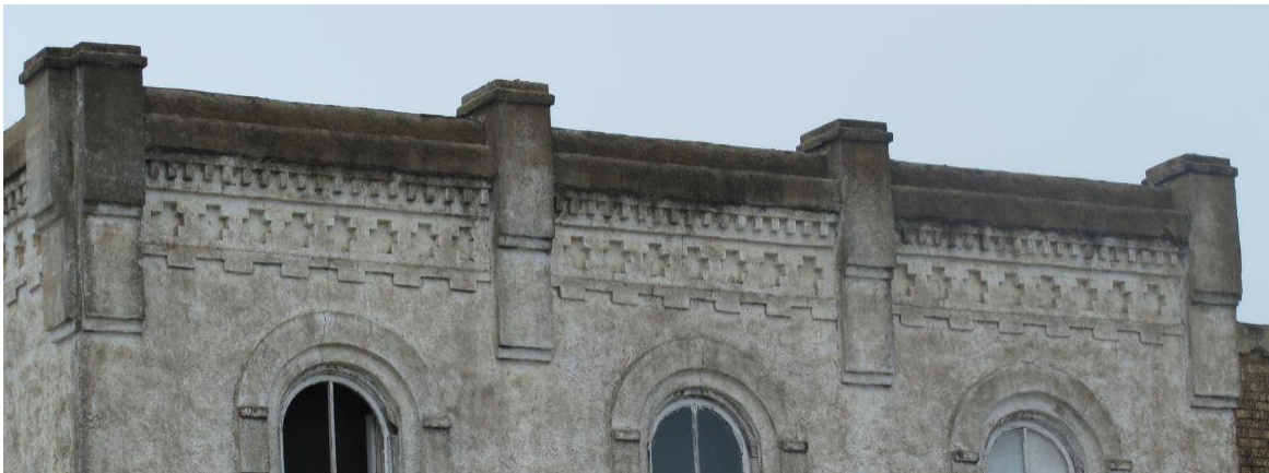
Figure 11: Image of the façade's parapet as it looks today. East elevation.
