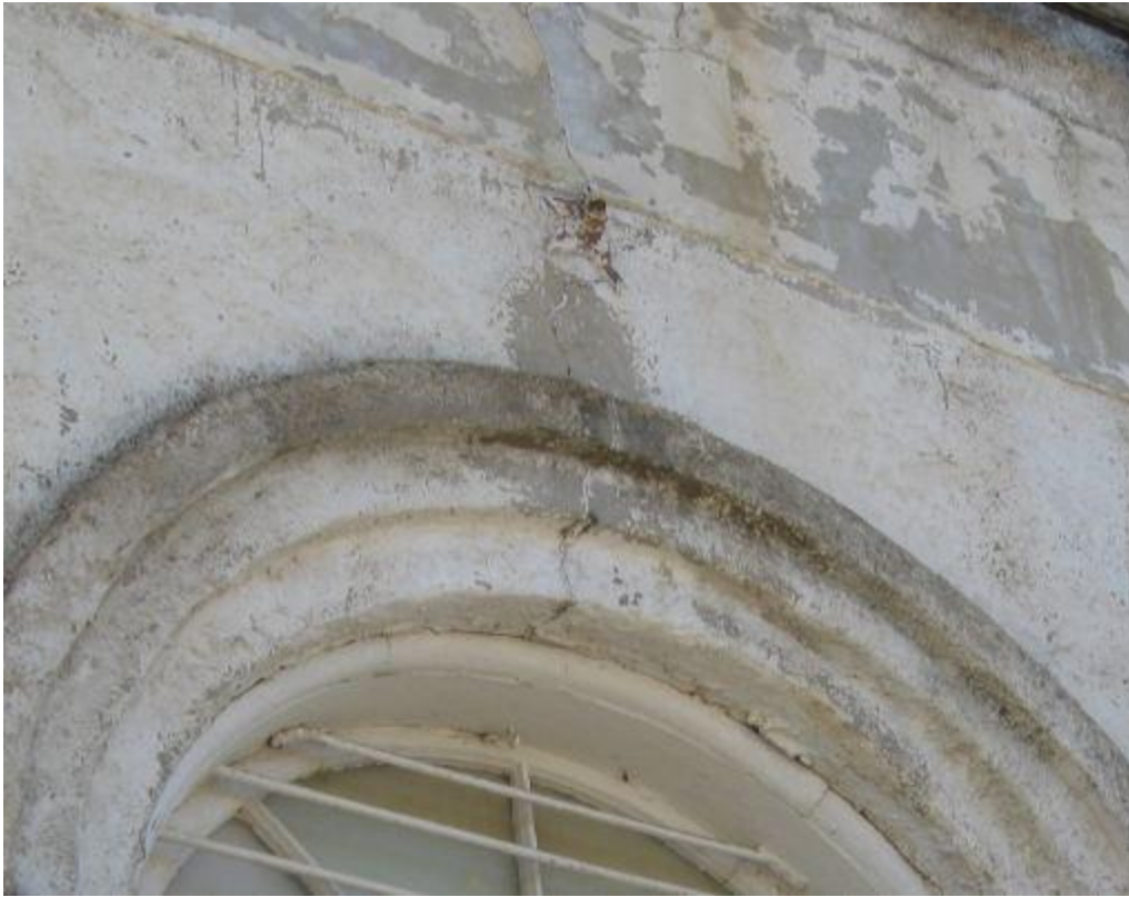
Figure 14: Star-shaped tie above the center opening. East elevation.
