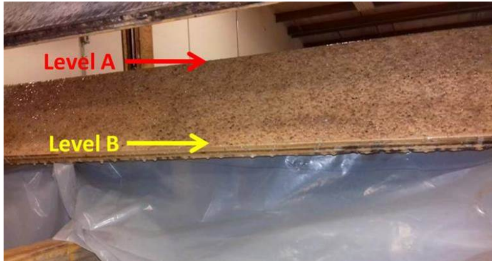
Figure 5.7: The two tested tail water levels, looking from inside the inlet.
