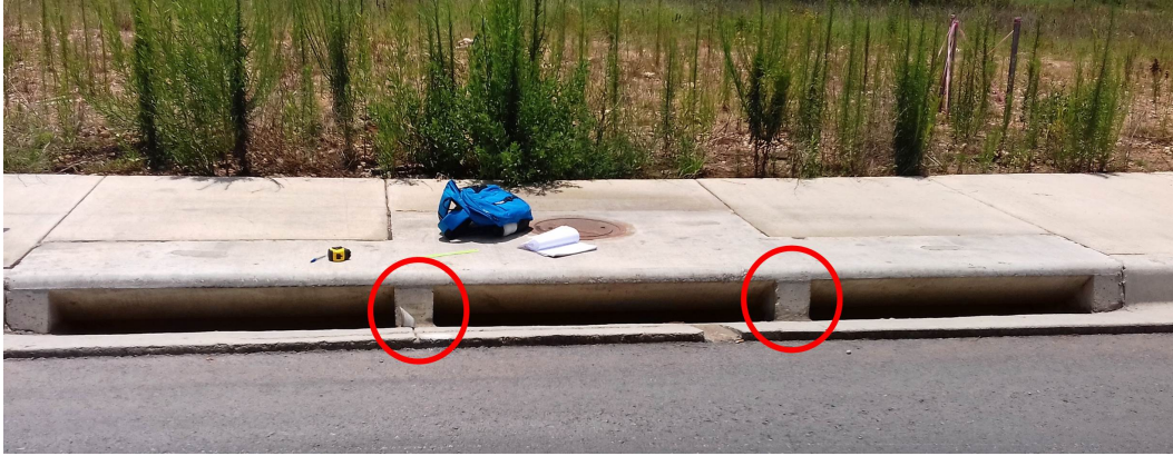
Figure 5.3: 15-ft PCO inlet with two slab supports highlighted.
