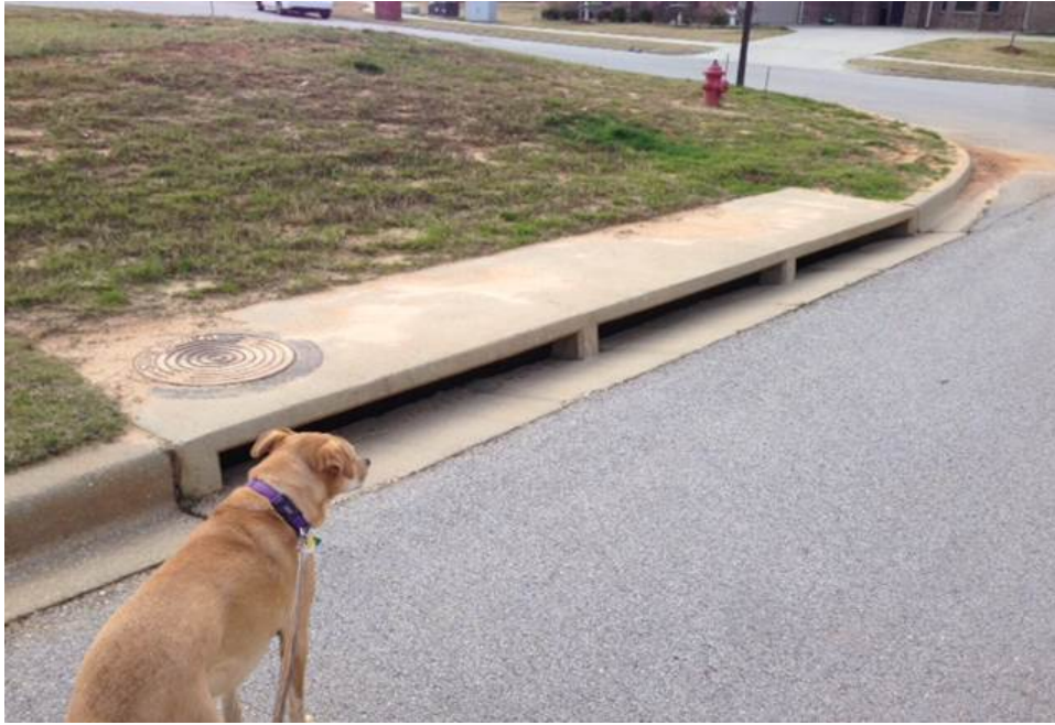
Figure 1.1: 15-ft curb-opening inlet.
