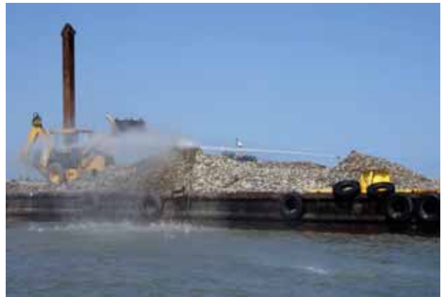
Oyster shells are blown into Copano Bay from a barge in The Nature Conservancy's oyster-reef restoration pilot project. Photo credit Mark Dumesnil/The Nature Conservancy
