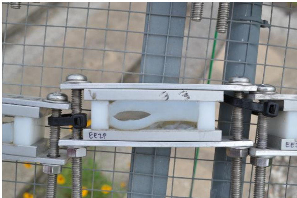
Figure 41: Specimen DRP1014-EE2P Partial Cohesive Failure After 4 Months in Extension
