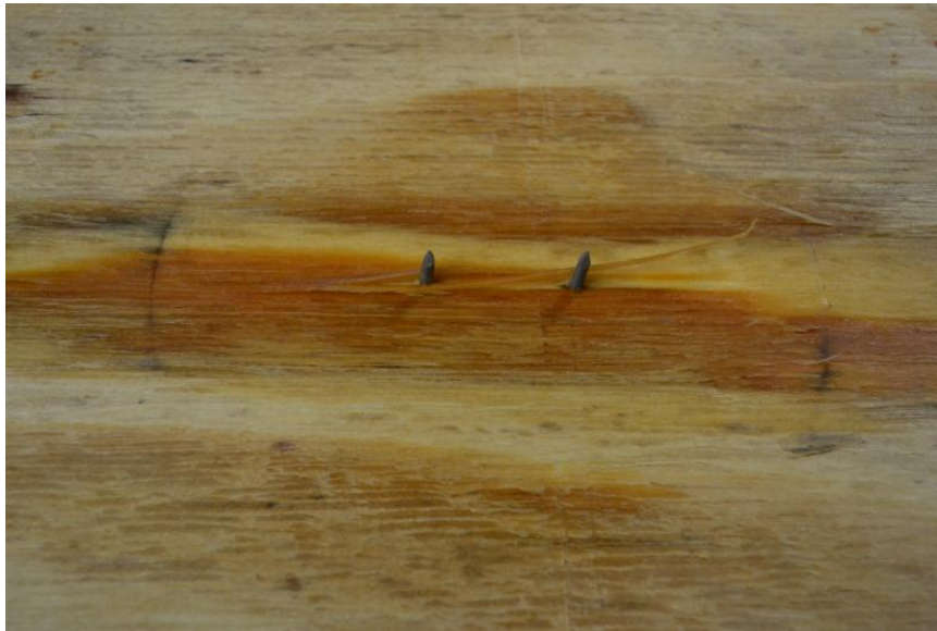
Figure 26: Significantly Saturated Underside of Plywood of Specimen DRP1009-03-A
