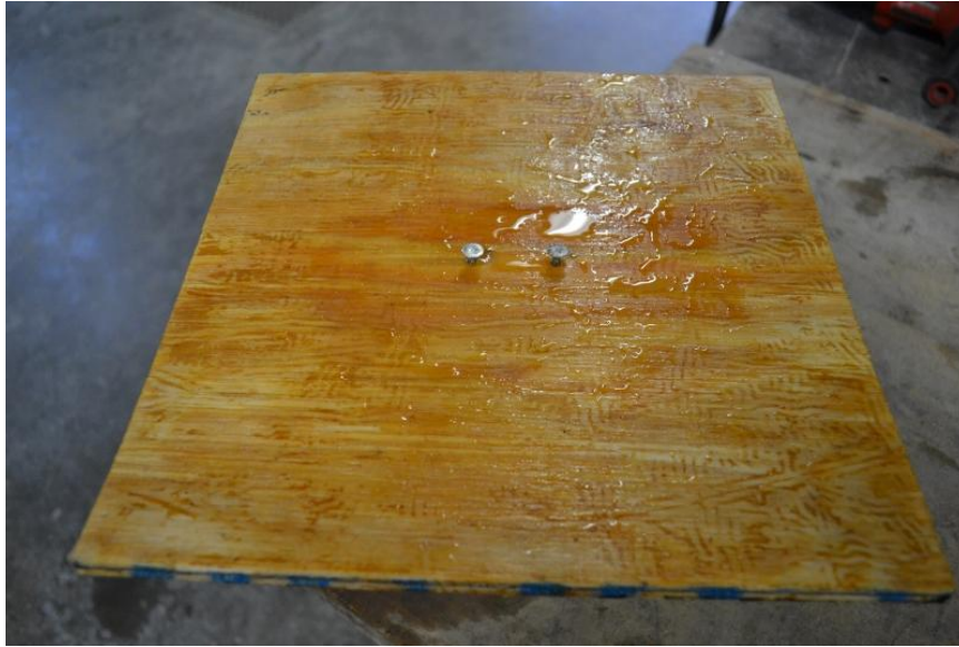
Figure 27: Significant Water Penetration Underneath Specimen DRP1009-06-B, a Self-adhered Membrane
