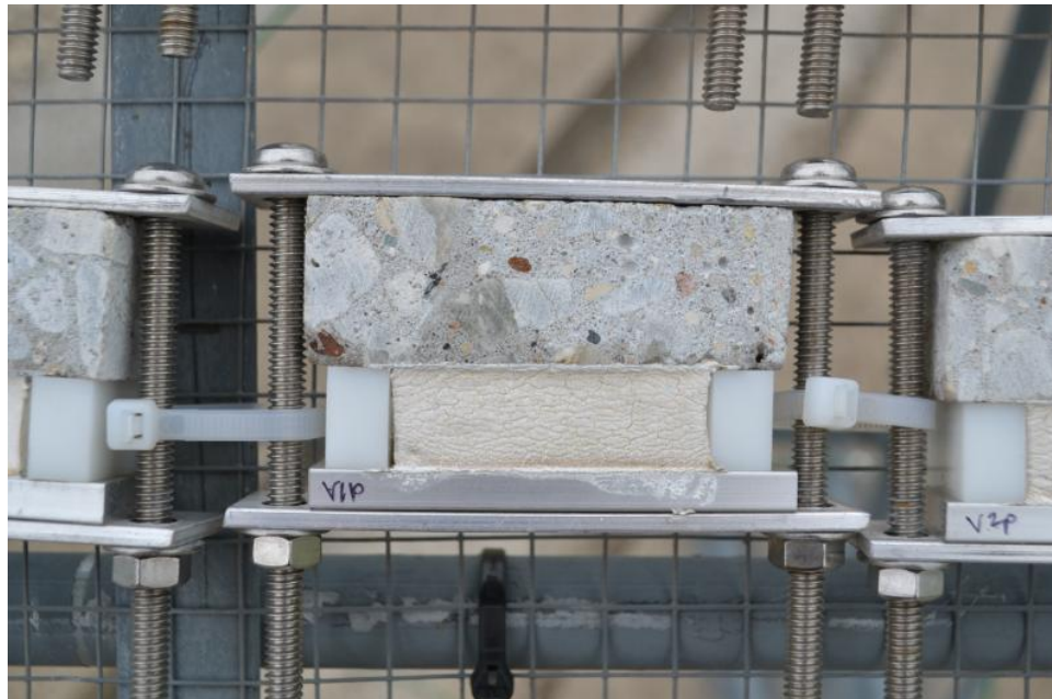
Figure 40: Specimen DRP1014-V1P Crazing After 4 Months in Extension
