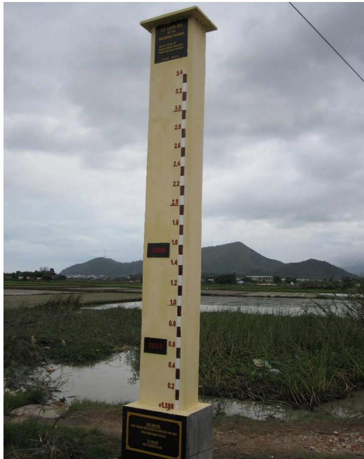
Figure 7.4: Pillar to Measure Flood Depth with Historical Flood Level Marks
