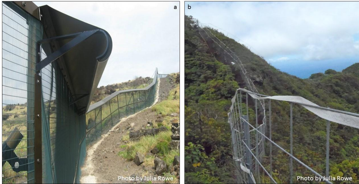
Figure 4.3. (a) Predator-proof fence at Ka‘ena Point, O‘ahu, HI, and (b) ungulate-proof fence in Upper Limahuli, Kaua‘i, HI.
