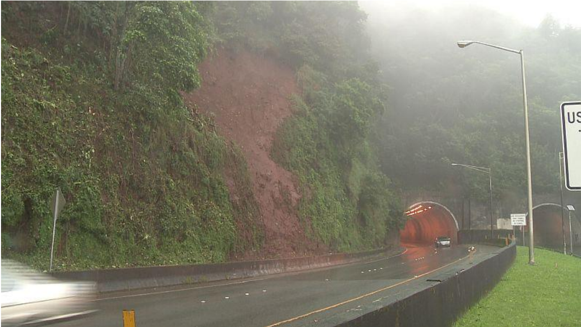
FIGURE 3.11 February 2014 landslide on Pali Highway
