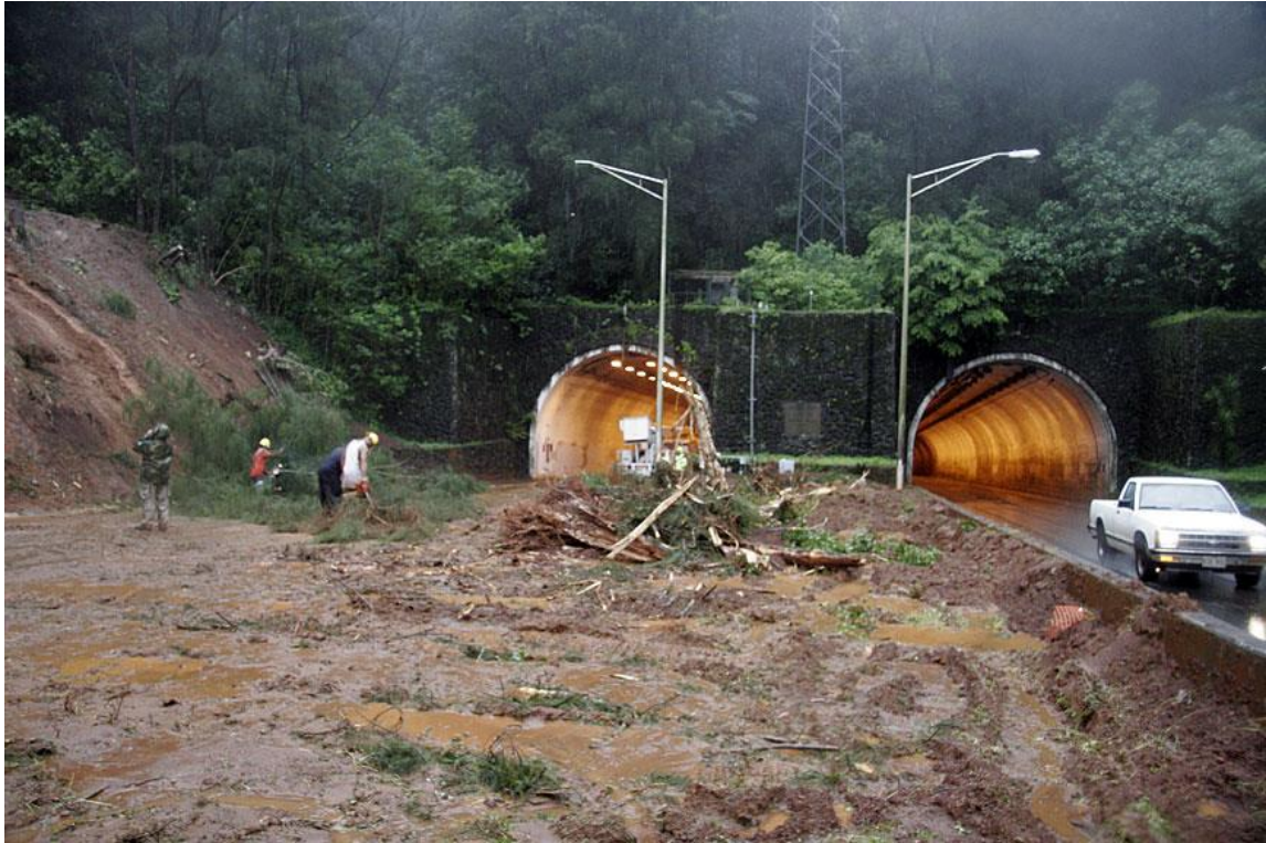
FIGURE 3.9 November 1, 2006 landslide on Pali Highway (Honolulu Star Bulletin, 2006)
