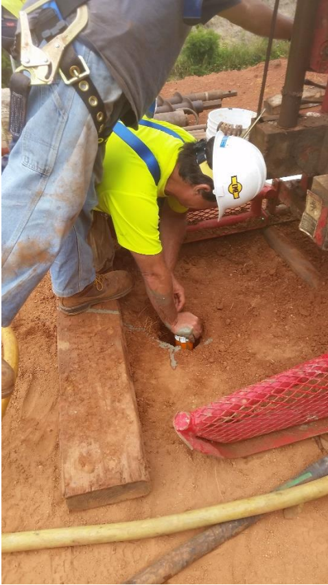
FIGURE 4.1 Installation of inclinometer casing
