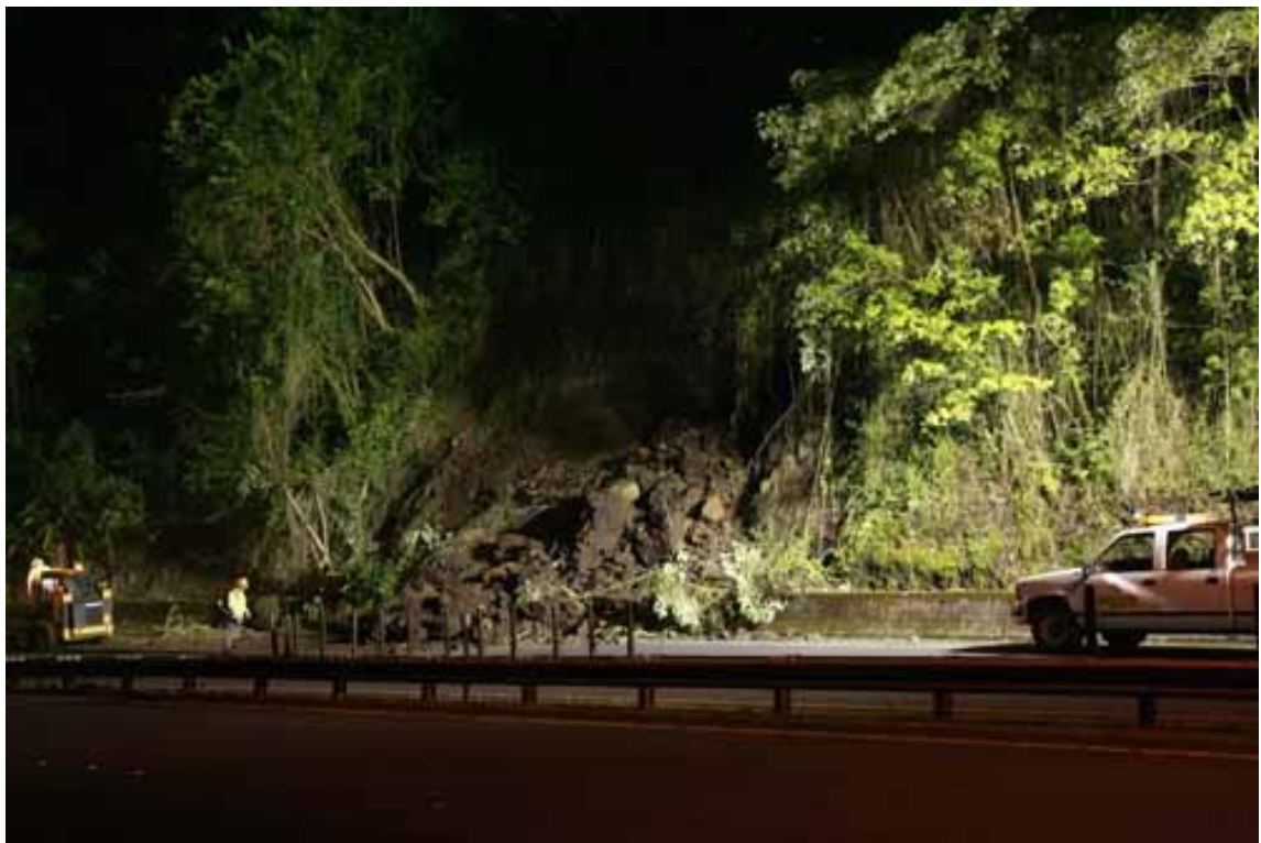
FIGURE 3.10 February 28, 2011 landslide on Pali Highway (Honolulu Star Advertiser, 2011)
