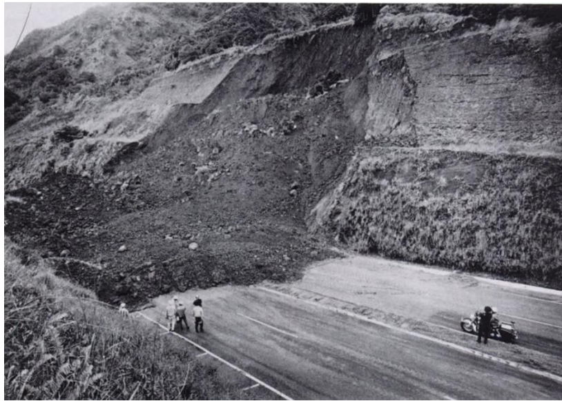
FIGURE 3.7 August 1967 landslide on Pali Highway at the same location as above (from Macdonald et al., 1983)
