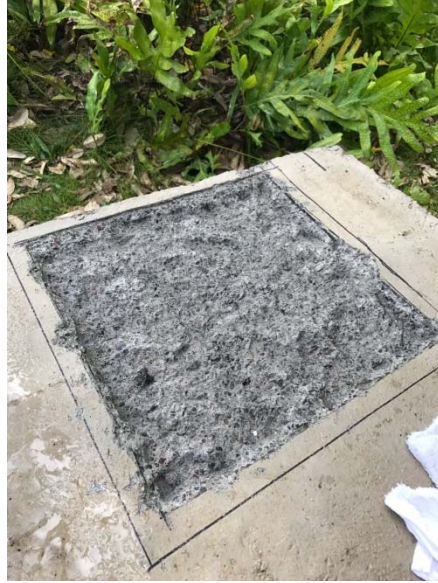
Figure 4-22 Surface preparation before mixing
