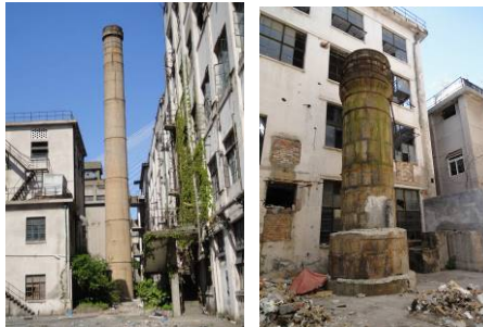
Fig3.16 Chimney 1 and 2 in Shanghai Chemical Factory 58
