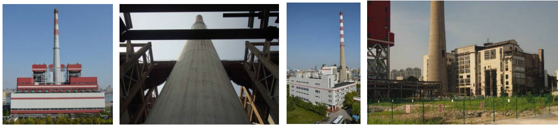
Fig3.17 Chimney 1-1,1-2,1-3 and 2 in Power Plant 59
