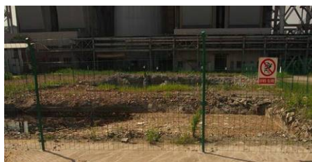
Fig3.18 Pump room underground space in Power Plant 60
