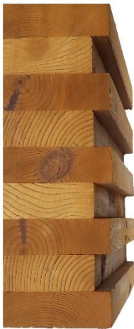
Figure 8.34 Brettstapel Construction
