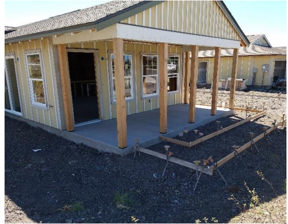
Figure 5.3: Kamakoa Nui Home, Under Construction, 2017
