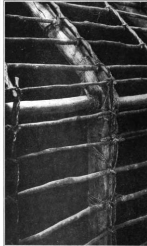
Figure 2.4: Hale Pili Timber Posts, Rafters and Purlins
