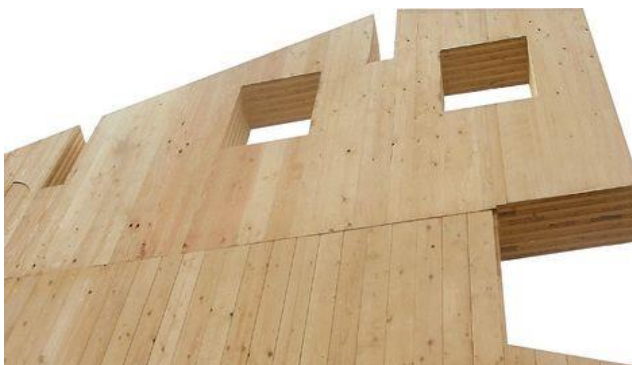
Figure 8.39: MHM Wall Structure
