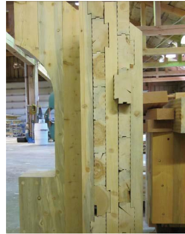
Figure 8.32: ICLT Panel
