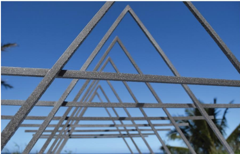
Figure 9.2: Pre-Cast Concrete Structure
