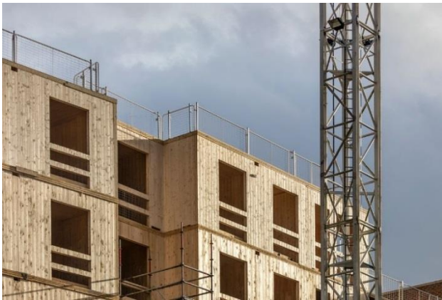
Figure 8.31: Dalston Lane, under construction 2016
