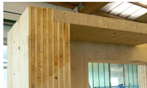
Figure 8.35 Hundegger PHE (Brettstapel) Roof Panel
