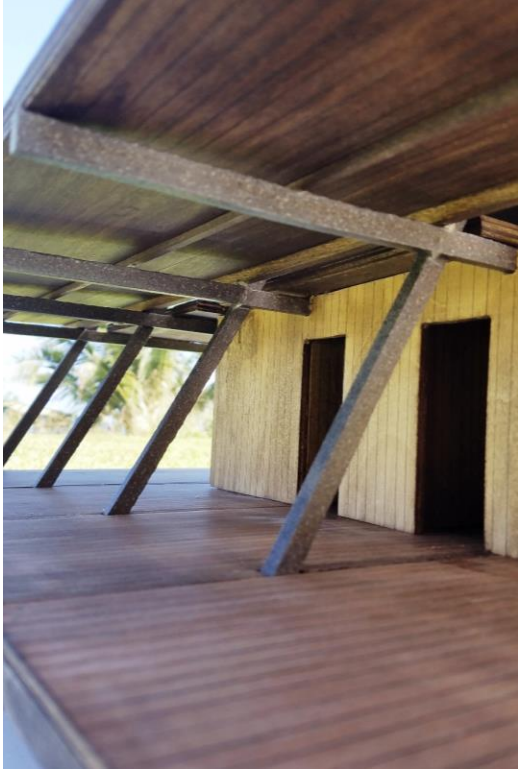
Figure 9.7: Thermally Modified Lanai Panels and Interior Walls
