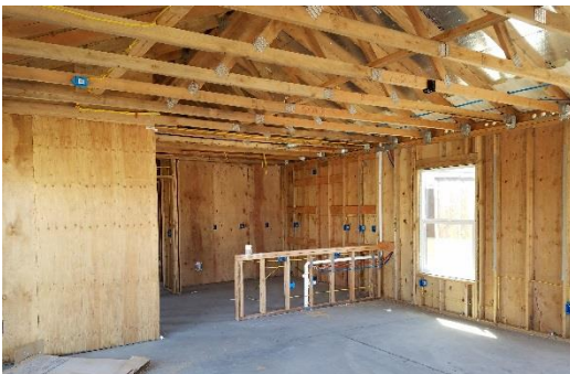
Figure 5.5: Kamakoa Nui, under construction 2017
