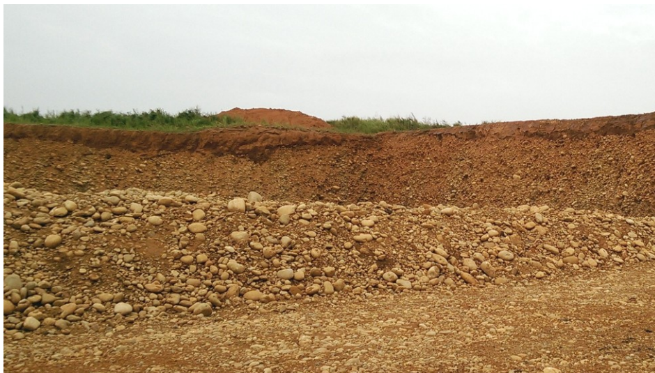
Figure 4.3. Red topsoil of the Dadu Plateau exposed at a construction site.
