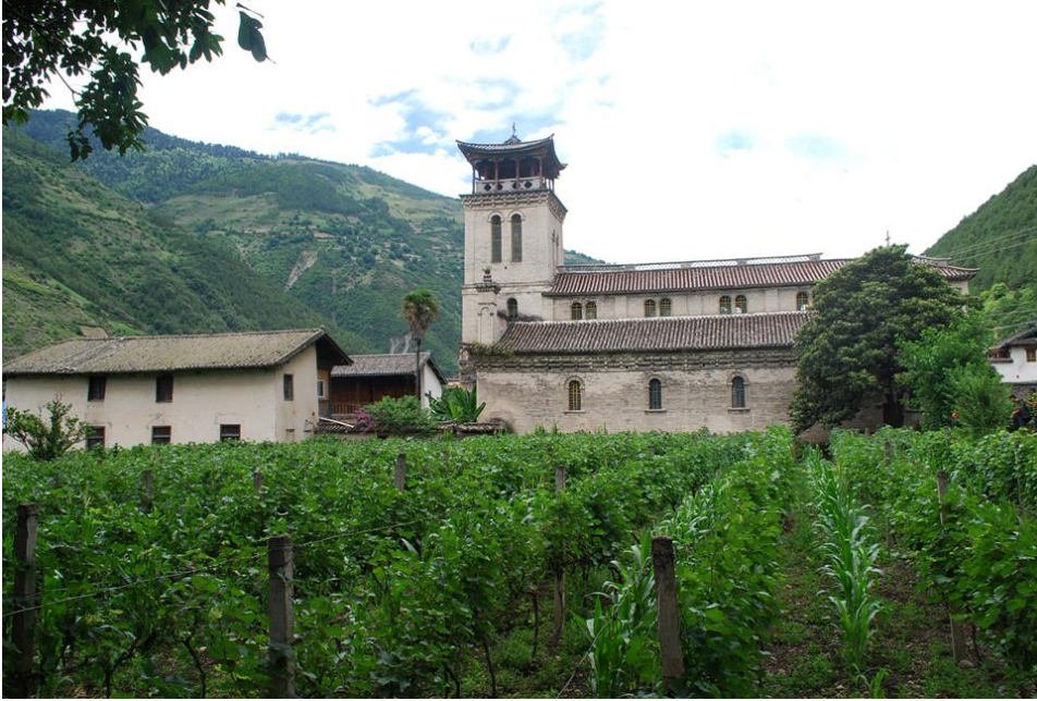
Figure 11. Cizhong church built in 1909. The Cabernet Sauvignon vineyards were planted in recent years by the Deqin County agricultural bureau.
