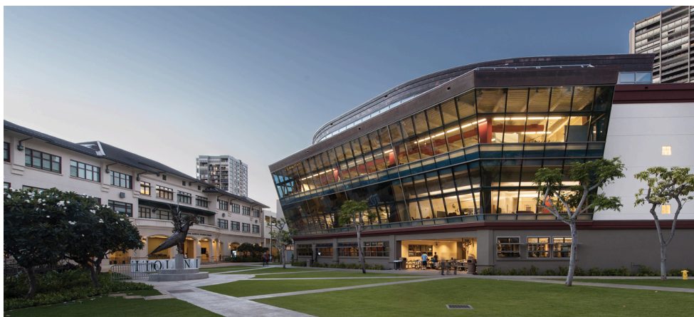
Figure 2.5: Sullivan Center, view of large glass façade (Photo from G70 Design website, http://g70.design/project/iolani-school-sullivan-center/ )
