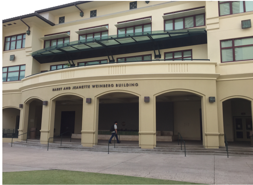
Figure 2.1: View of Weinberg Building looking makai (photo by author)
