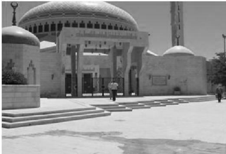
Image 3. Photo of grand mosque with no ramp.
