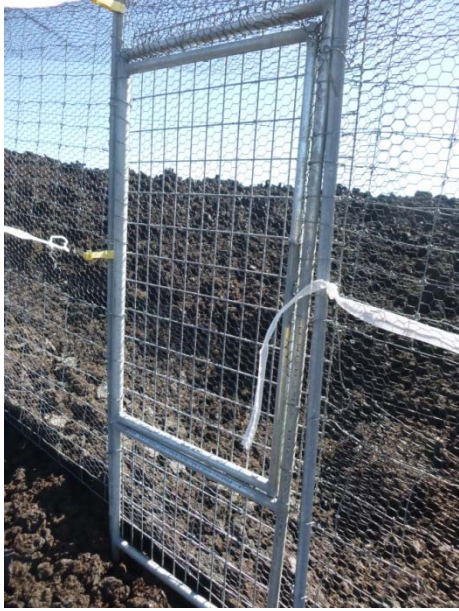
Figure 26 Attaching the gate frame to the T posts
