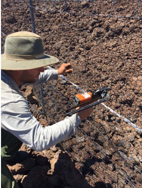
Figure 18 Attaching mesh to hog wire using hog rings
