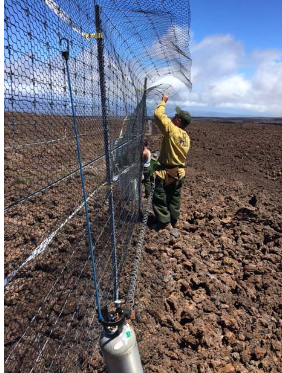
Figure 19 Using the CO 2 powered hog ring tool
