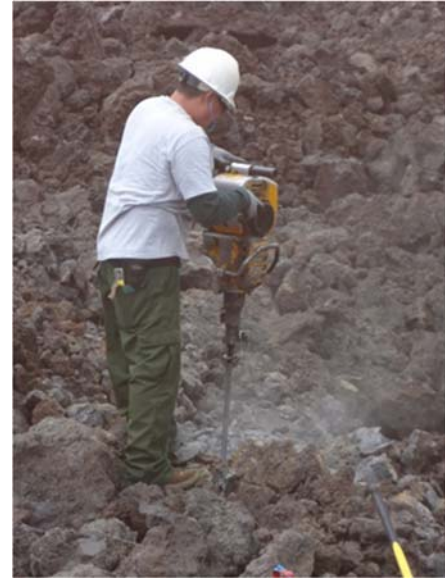
Figure 14 Drilling holes to sink the posts
