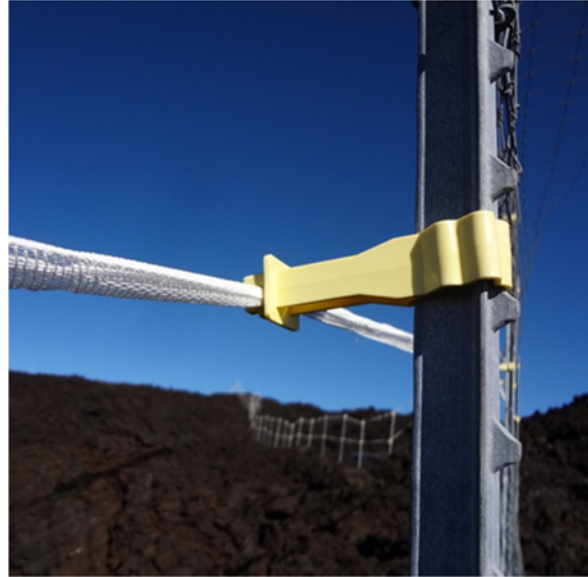
Figure 16 T-post insulator to reduce friction
