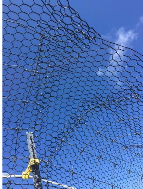
Figure 23 Splicing in mesh as needed
