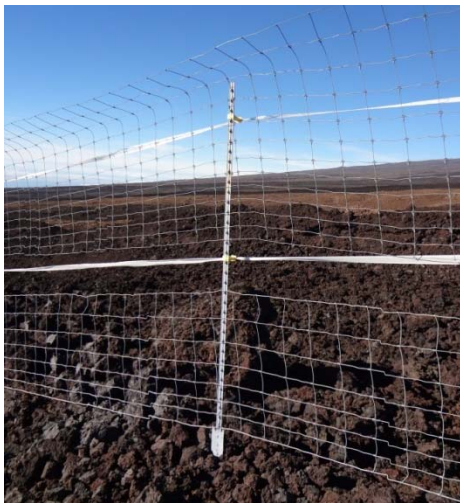
Figure 17 Two heights of hog wire for stability
