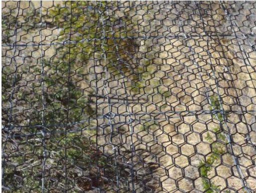
Figure 7 PVC coated hexagonal mesh
