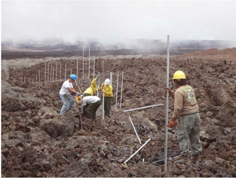
Figure 13 Lining up and setting the posts
