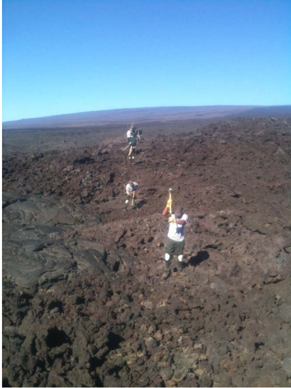
Figure 12 Fence crew pulverizing the route
