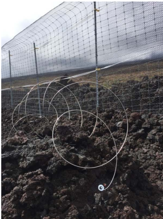
Figure 28 Smooth wire coiled on high spot
