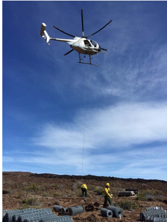
Figure 31 Sling loading fence materials to the site
