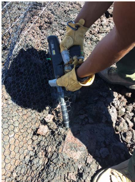
Figure 21 Attaching mesh skirt to surface using nail gun
