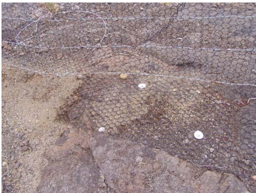
Figure 8 HAVO design modification; skirted affixed to surface
