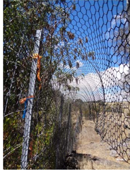
Figure 11 Sheep wire did not support arc
