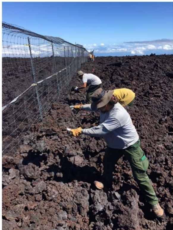
Figure 20 Stacking rocks to secure the mesh skirt
