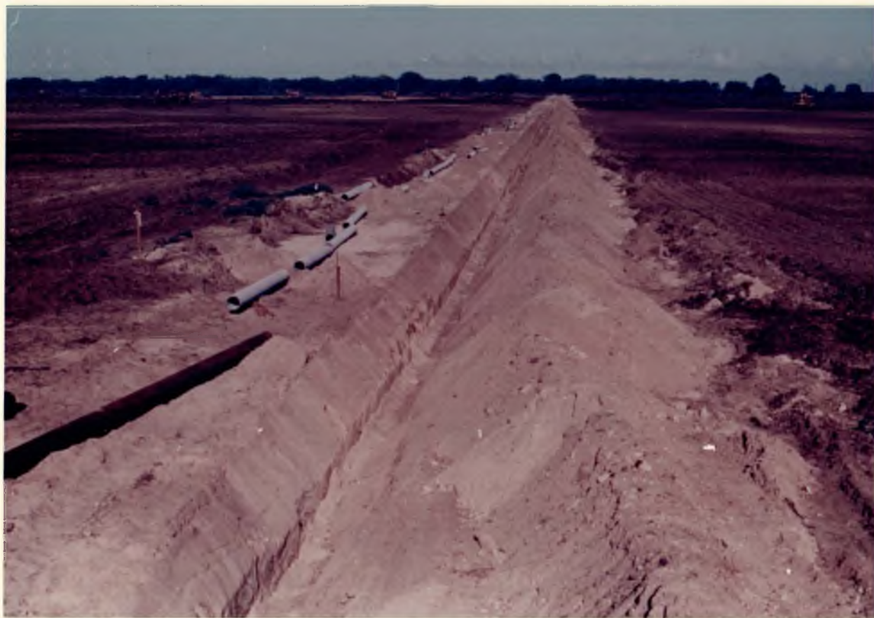
FIGURE 4. RECLAMATION OF CALCAREOUS SOIL (CATANO SAND). NOTE INCORPORATION OF BAGASSE AND USE OF TILES.
