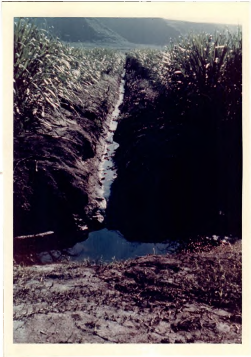
FIGURE 5. "BUCKET" TRENCH UTILIZED FOR DRAINAGE.
