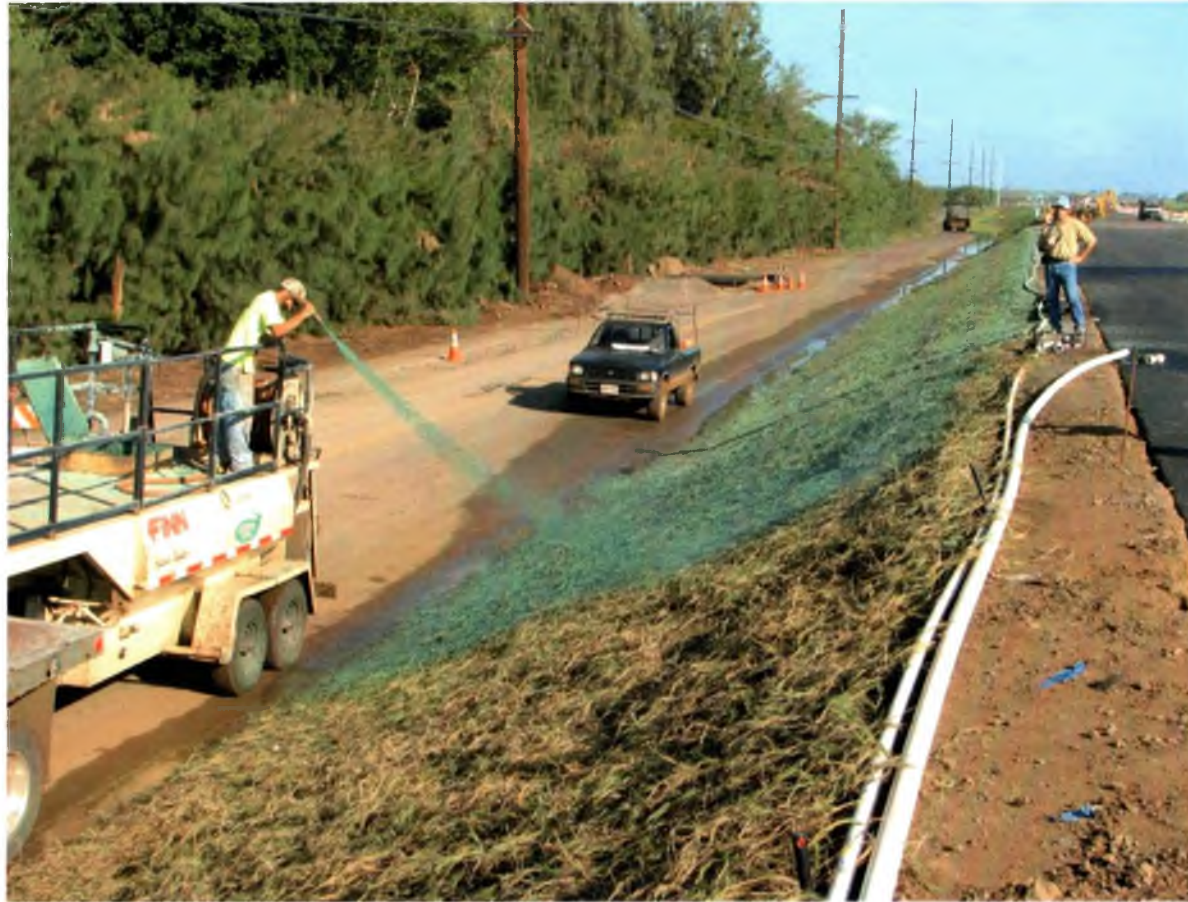
Figure 3.1. Hydromulch capping of untreated S. virginicus stem cuttings along the Mokulele Highway near Kihei, Maui (February 2008). Although this method of planting has already been employed in the field, studies on rooting success need to be conducted in order to efficiently utilize planting materials.
