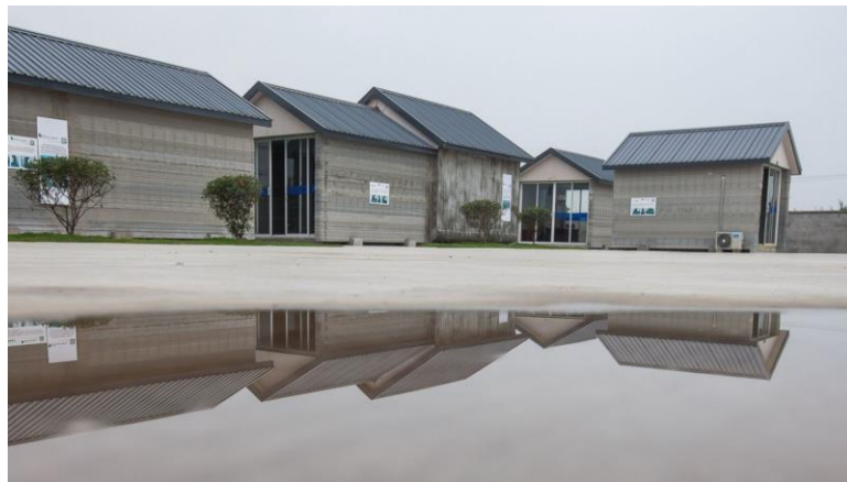
Figure 4.5– Photo showing ten homes created by a 3D printer in twenty-four hours by a company called Winsun 121
