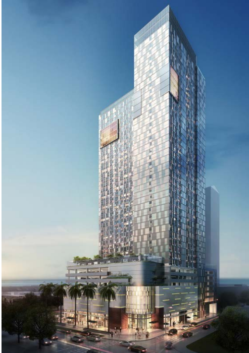
Figure 94: Ke Kilohana Condominium High-Rise
