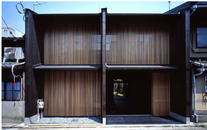
Figure 28: A House With 3 Walls
