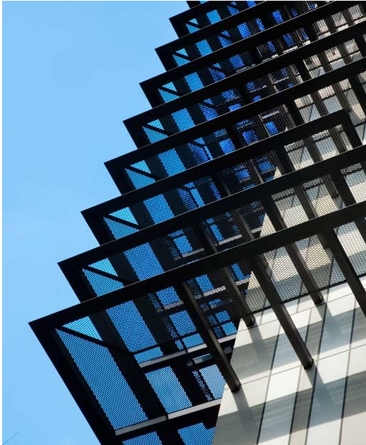
Figure 61: Building Shading Device
