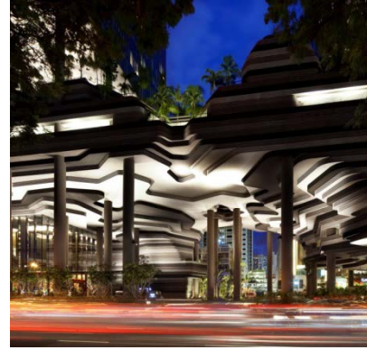
Figure 82: Organic Formwork of the Facade and Ceiling
