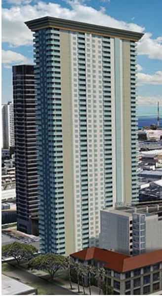
Figure 92: 801 South Street Apartments High-Rise
