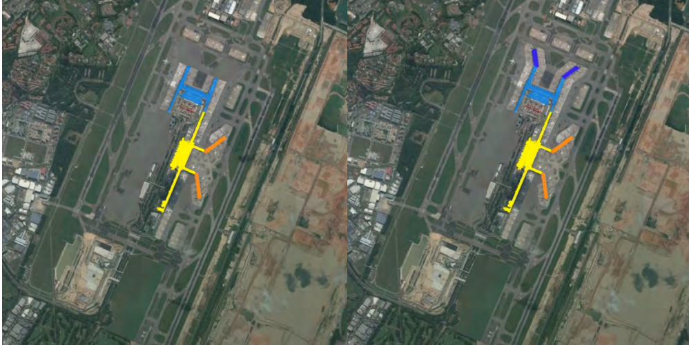
Figure 7. Terminal 1 Extension, added onto two piers of Terminal 1, just like Terminal 2 Expansion/Terminal 2.
