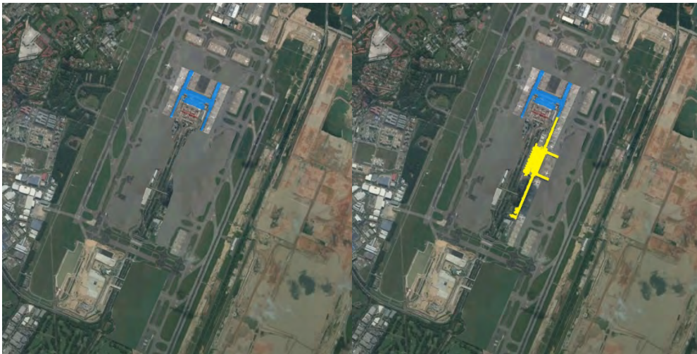
Figure 5. Terminal 2 built upon the southeast pier of Terminal 1.
