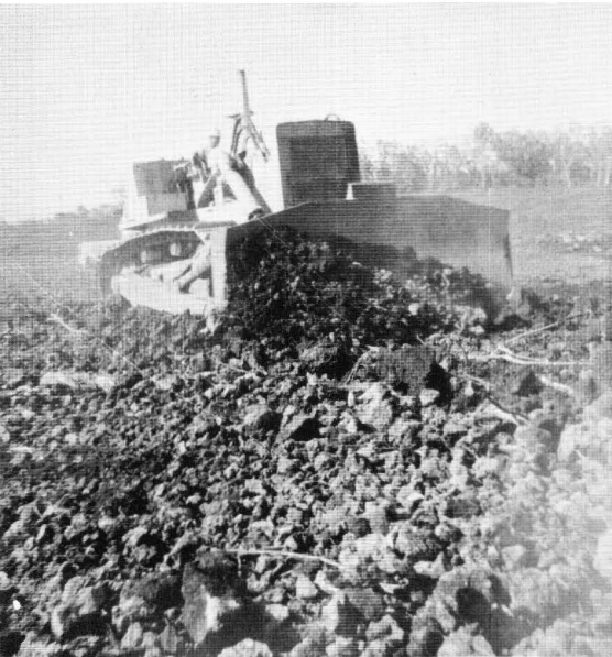
Smoothing out and burying rocks prior to rolling.
