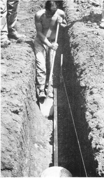
Fig. 43 (left). A mark on the stick lying in the trench bottom indicates the site of the next joint. An excavation is made here which is filled with mortar. On placing the pipe, good contact should be established between the groove or bell end and the mortar in the excavation as this will become the bottom section of the mortar band surrounding the joint. (See fig. 7.)
