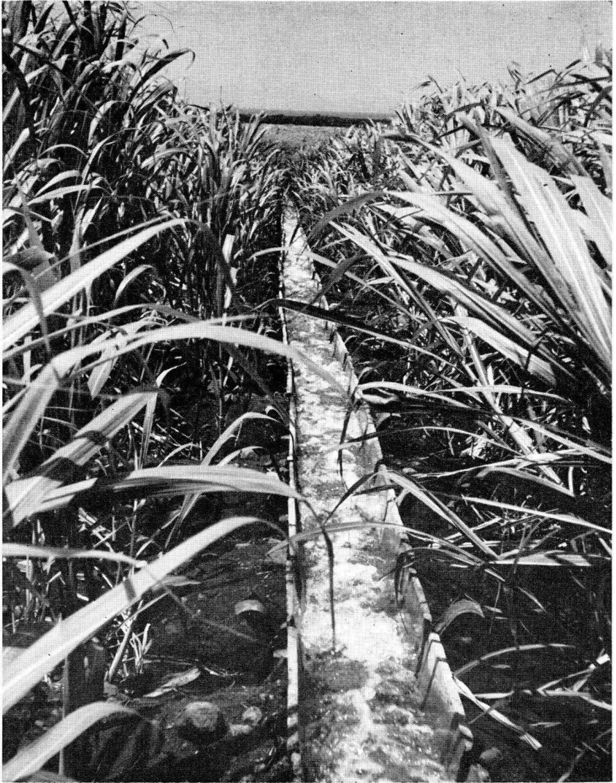
Fig. 2. The high velocity in concrete flumes on steep slopes makes it difficult to intercept water for diversion into the furrows.
