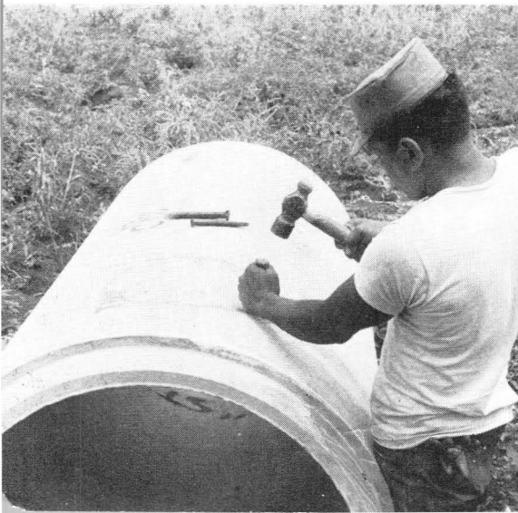
Fig. 49. Before installing standpipes, holes for pipe inlets are chipped out.
