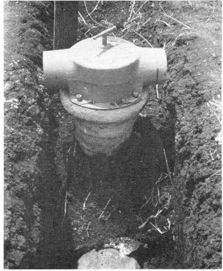
Fig. 27. A furrow valve installed on top of a bell at the end of a line. A coupling is welded on to either outlet to which surface pipe is attached.
