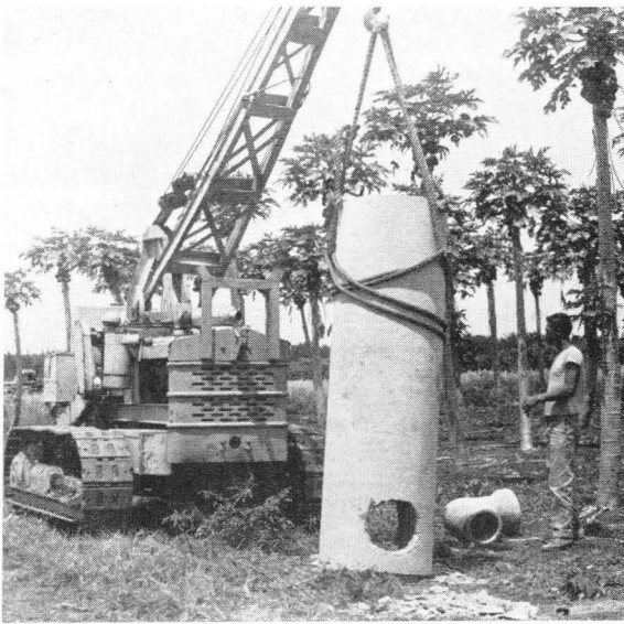
Fig. 50. The standpipe is now ready for installation. The margin below the pipe inlets allows the standpipe to be set in a concrete footing.
