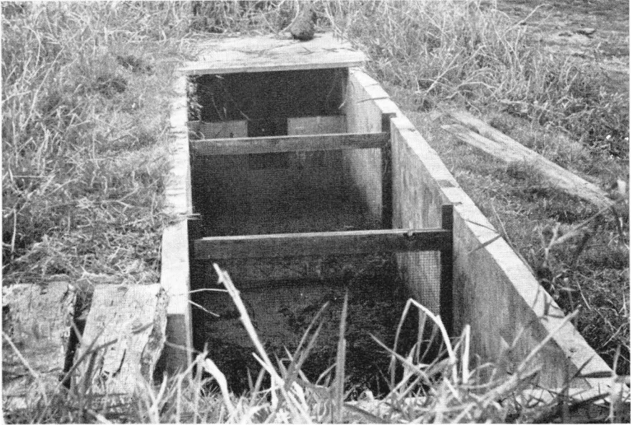
Fig. 36. Water is taken from a ditch (left) and discharged via a rectangular weir into buried concrete pipe. This weir requires an elaborate approach channel, as shown.
