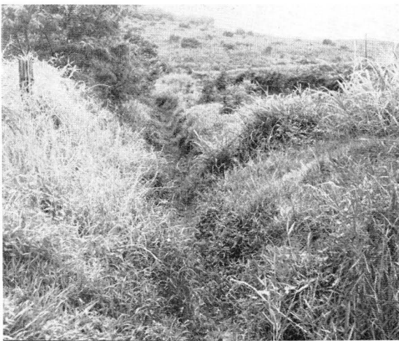
Fig. 5. Unlined irrigation ditches require weed control.
