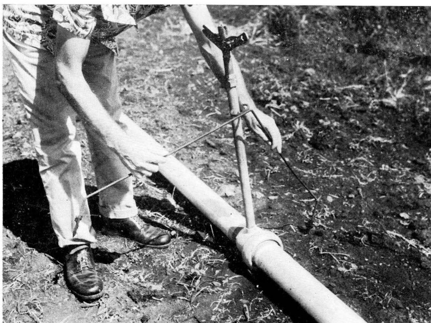
Figure 3. Construction and installation of type A riser support.
