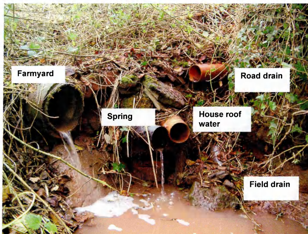
Plate 7.2 Piped discharges of runoff from multiple sources feeding into a headwater stream in the Kivernoll catchment.
