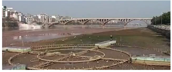
Figure 1: In (a) the demolition of a bridge Guangxi, China. The excavator in this picture was used to initiate some failure at one end of the bridge propagates through the structure. The figure shows the resulting periodic failure process, where the supporting columns fail sequentially causing the collapse of the bridge. An alternative view of this process is presented in (b).
