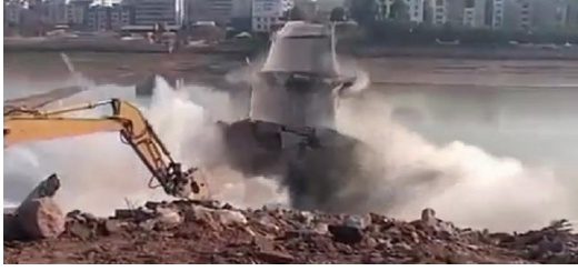
Figure 1: In (a) the demolition of a bridge Guangxi, China. The excavator in this picture was used to initiate some failure at one end of the bridge propagates through the structure. The figure shows the resulting periodic failure process, where the supporting columns fail sequentially causing the collapse of the bridge. An alternative view of this process is presented in (b).
