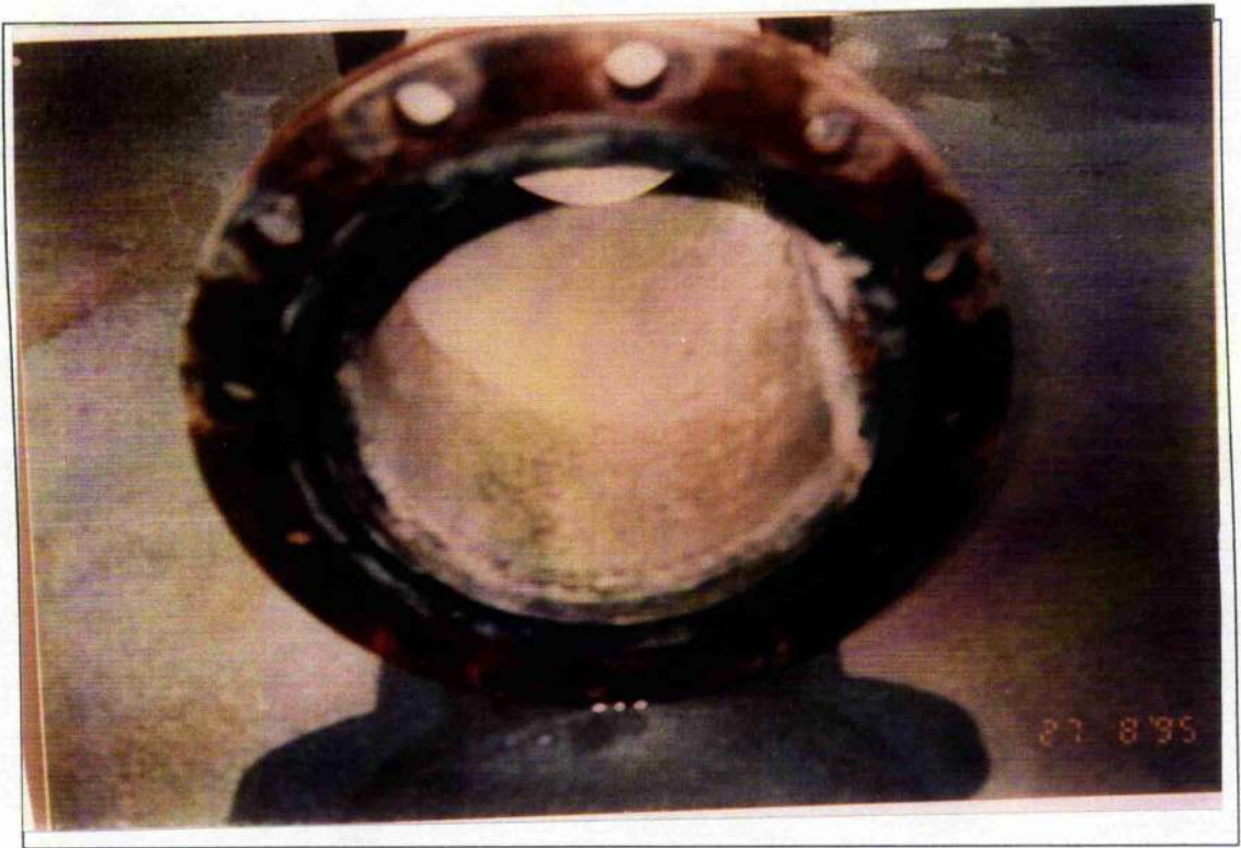
Figure 8.65: Specimen condition after the end of test 44
