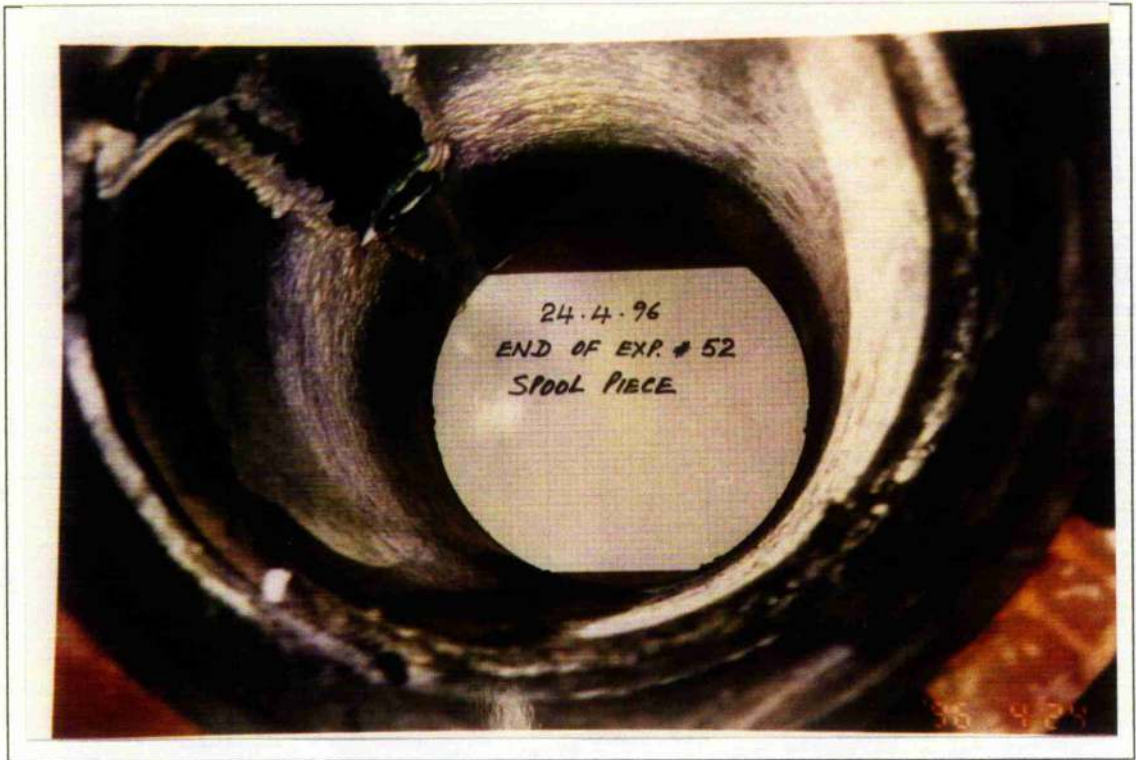
Figures 8.89: Spool condition at the end of test 52.
