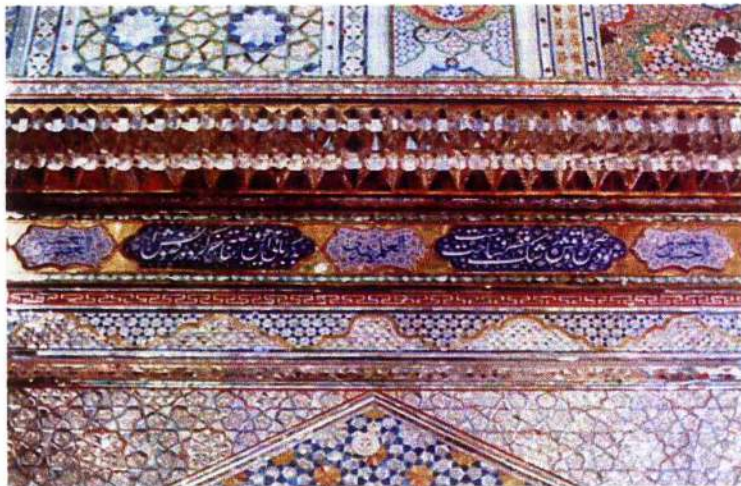
Image 35: Closer image of mirror - mosaic work on the edge of the wall. Shrine of Shah Chiragh, Shiraz.
