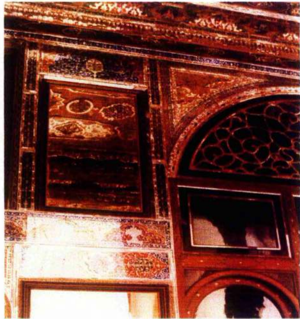
Image 49: Mirror - mosaic work in combination with coloured glass and woodwork on the wall. The house of Ghawam, Shiraz.
