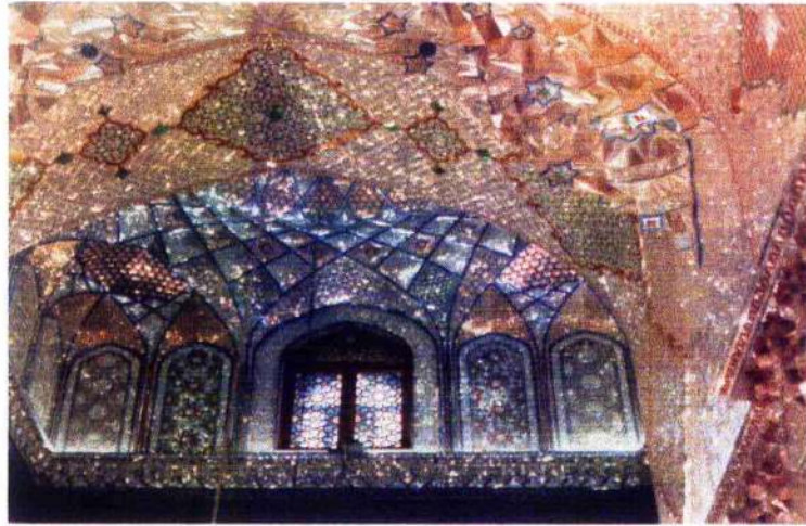
Image 39: Further example of mirror - mosaic work. Shrine of 'Ala al-din Husayn, Shiraz.
