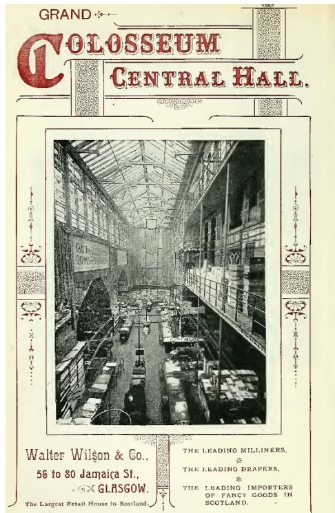
Figure 9: The Grand Hall and atrium of Wilson's Colosseum 57
