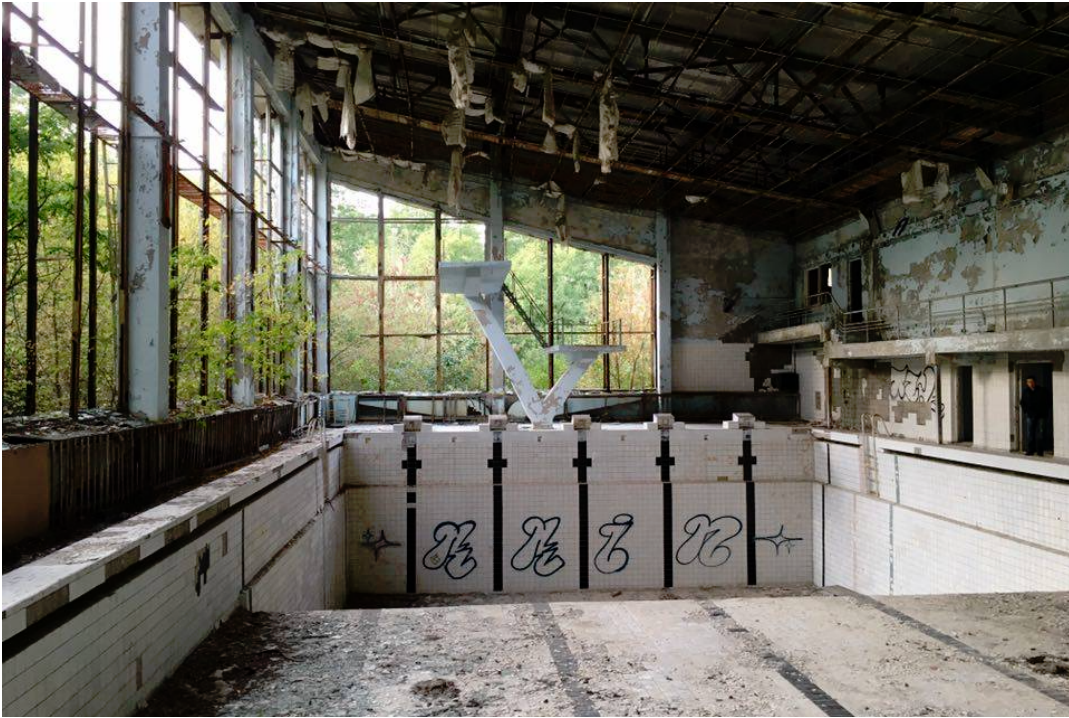
Figure 1.8: The swimming pool of the Cultural Palace (source: researcher's own photograph 2015)
