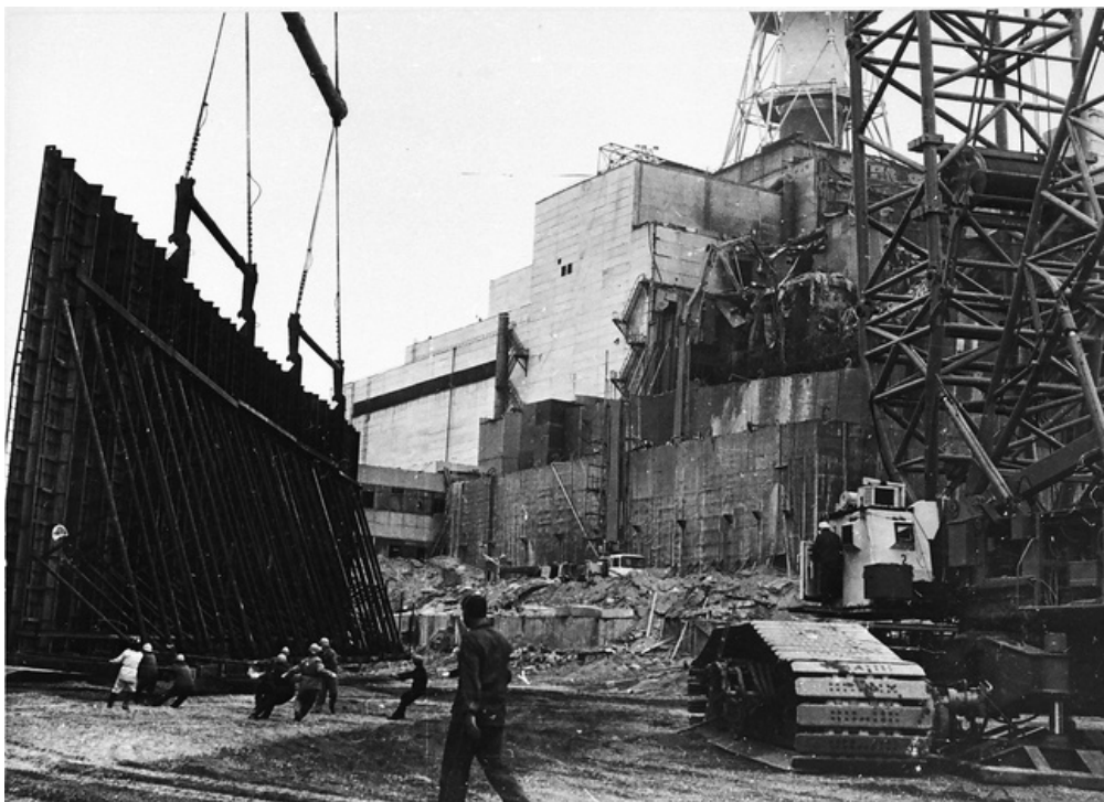
Figure 4.16: Construction work on the Sarcophagus (source: Kostin 2006)
