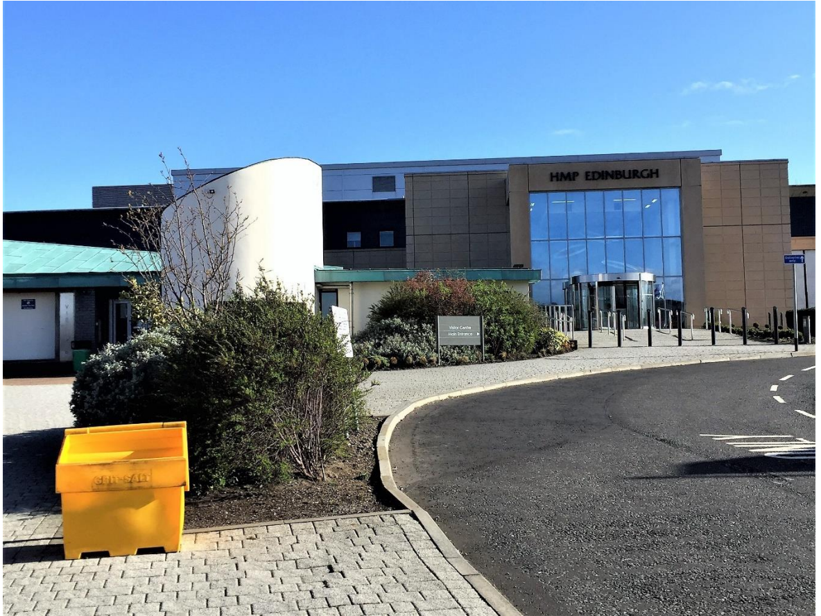
Figure 2: Photograph of exterior of HMP Edinburgh and the Visitors' Centre
