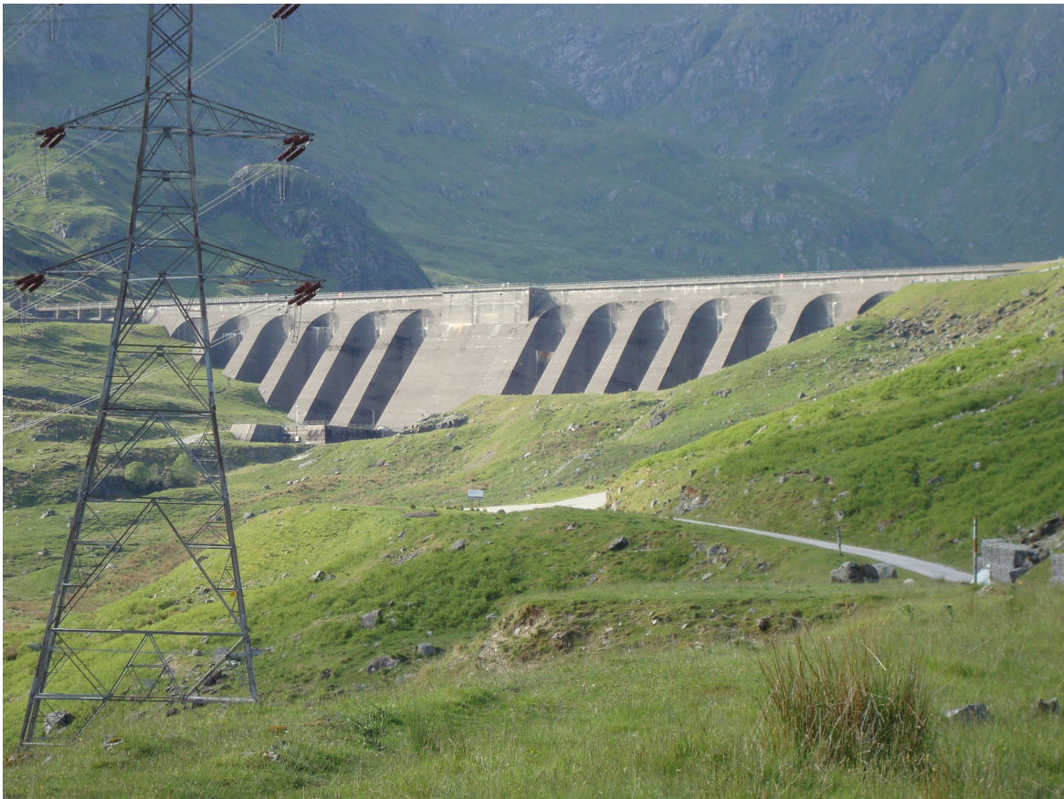
Fig. 6.6 The Cruachan pumped storage hydro-electric dam. This dam will be used to conduct a time-lapse gravity survey as the water level rises and falls.
