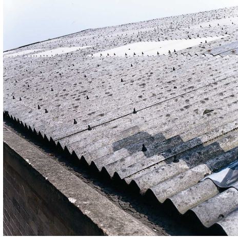
Figure 2-1: Asbestos cement roof cladding
