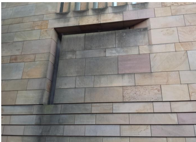
Figure 3-2: National Museums of Scotland; constructed using Clashach sandstone and emphasising the heterogeneity within the different beds of the quarry.
