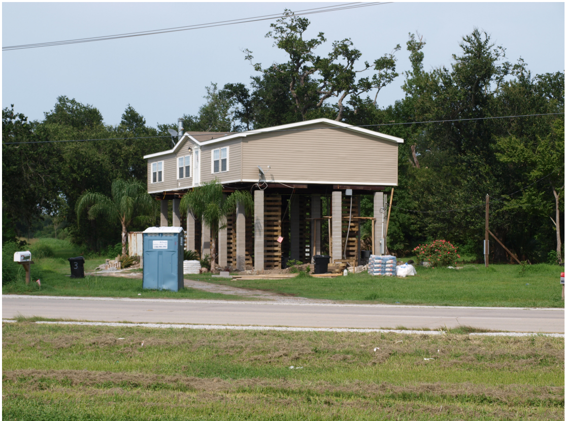
Image 10: House being raised on stilts.
