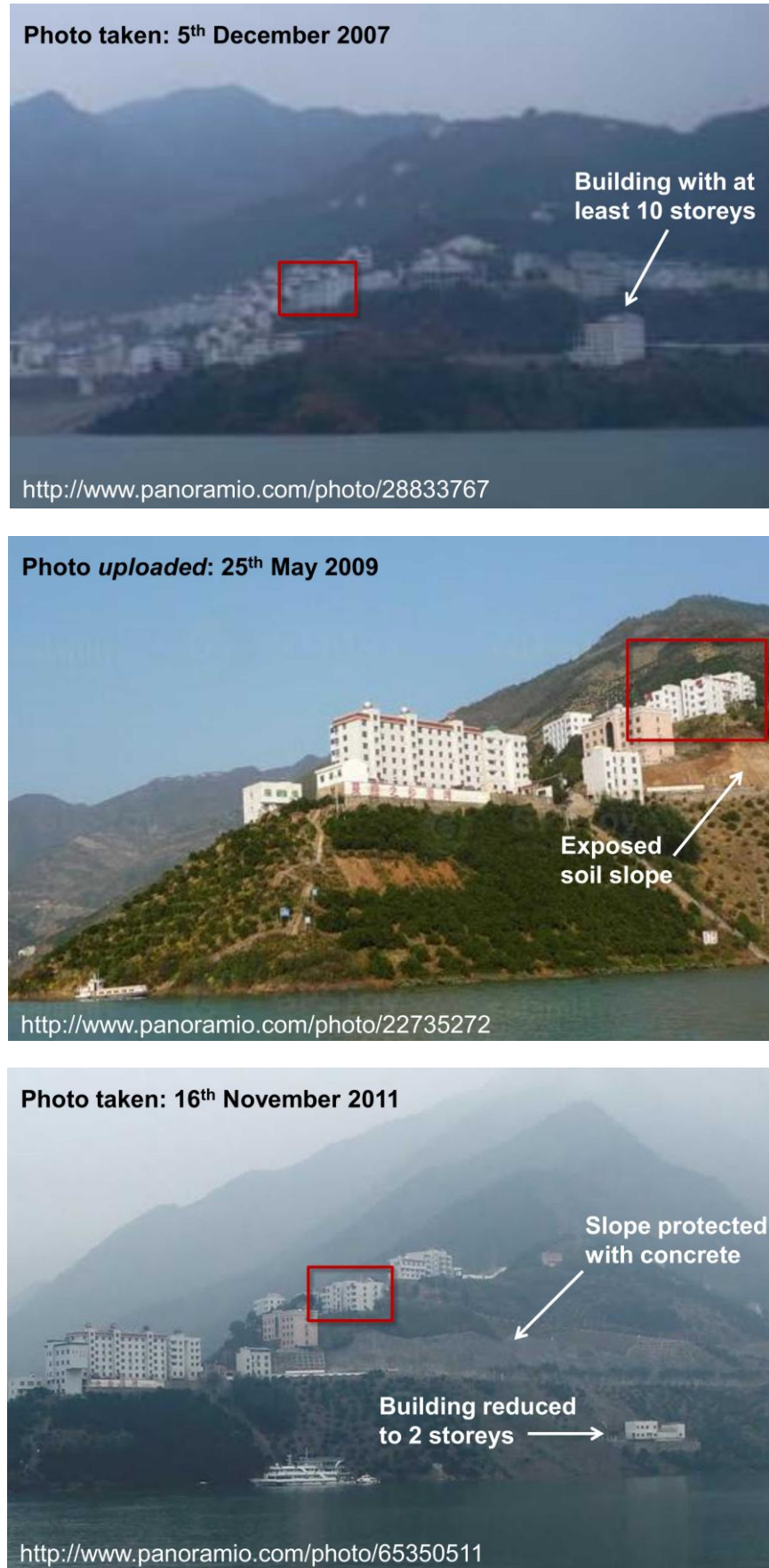
Figure 5-21: Online photos of the new riverbank instability area in three different years, from Panoramio & Google Maps. The red box highlights the same building to aid comparisons between images. The slope cutting above the road appears to have been reinforced by concrete and a tall building towards the base of the slope has been reduced in height, but not totally demolished.
