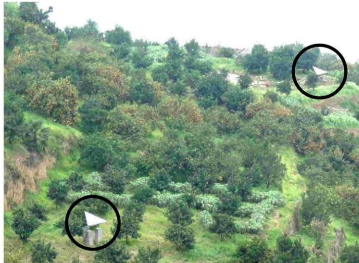
Figure A-1: Installed corner reflectors at the toe of the densely vegetated Shuping landslide. Edge lengths are approximately 1.5 m long.
