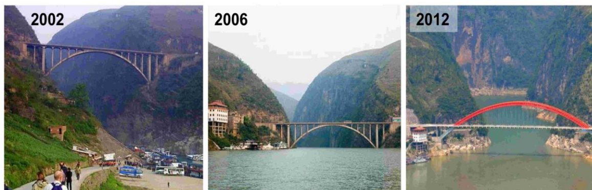
Figure 3-7: Impact of the Three Gorges reservoir impoundment on the Dragon Gate Bridge (31.1N, 109.9E). The bridge was overtopped by the reservoir, destroyed, and replaced by a higher bridge.
